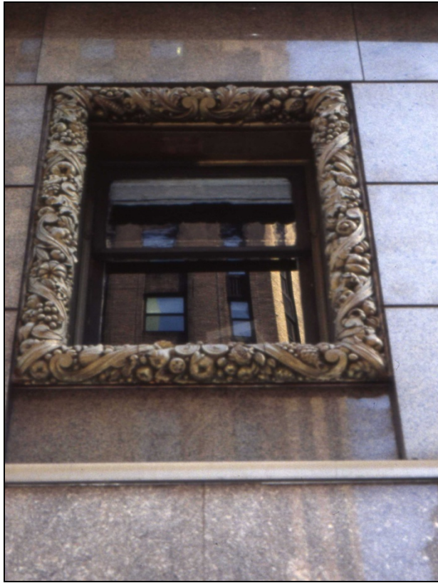
Window, second floor Photo: Mary Beth Betts, c. 2000
