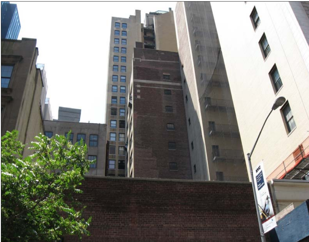
View from West 58 th Street, northeast corner of rear section Photo: Christopher D. Brazee, 2009
