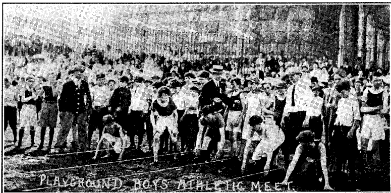
QUEENSBORO PARK PLAYGROUND STADIUM, FOOT OF EAST 59TH STREET, UNDER QUEENSBORO BRIDGE, JULY 4, 1912.
