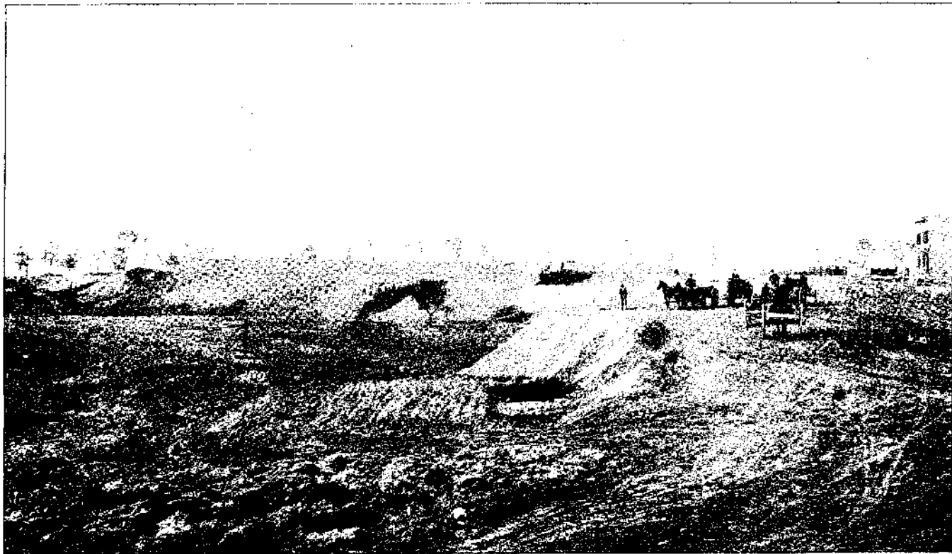
CONSTRUCTION OF BUFFALO AVENUE AND LINCOLN TERRACE.
