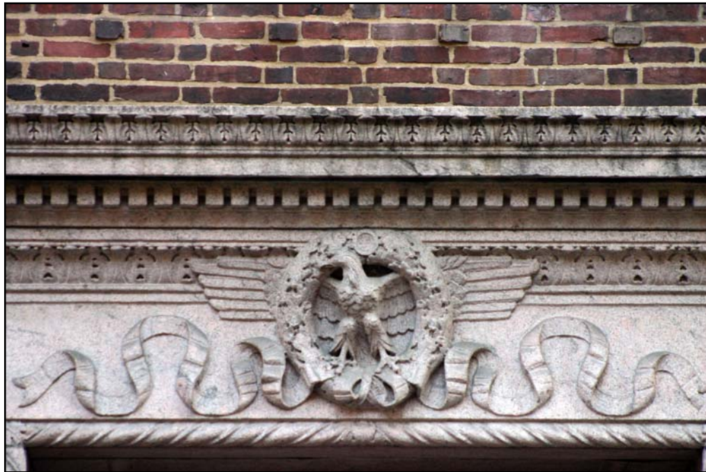
South Elevation: detail Photo by: Carl Forster
