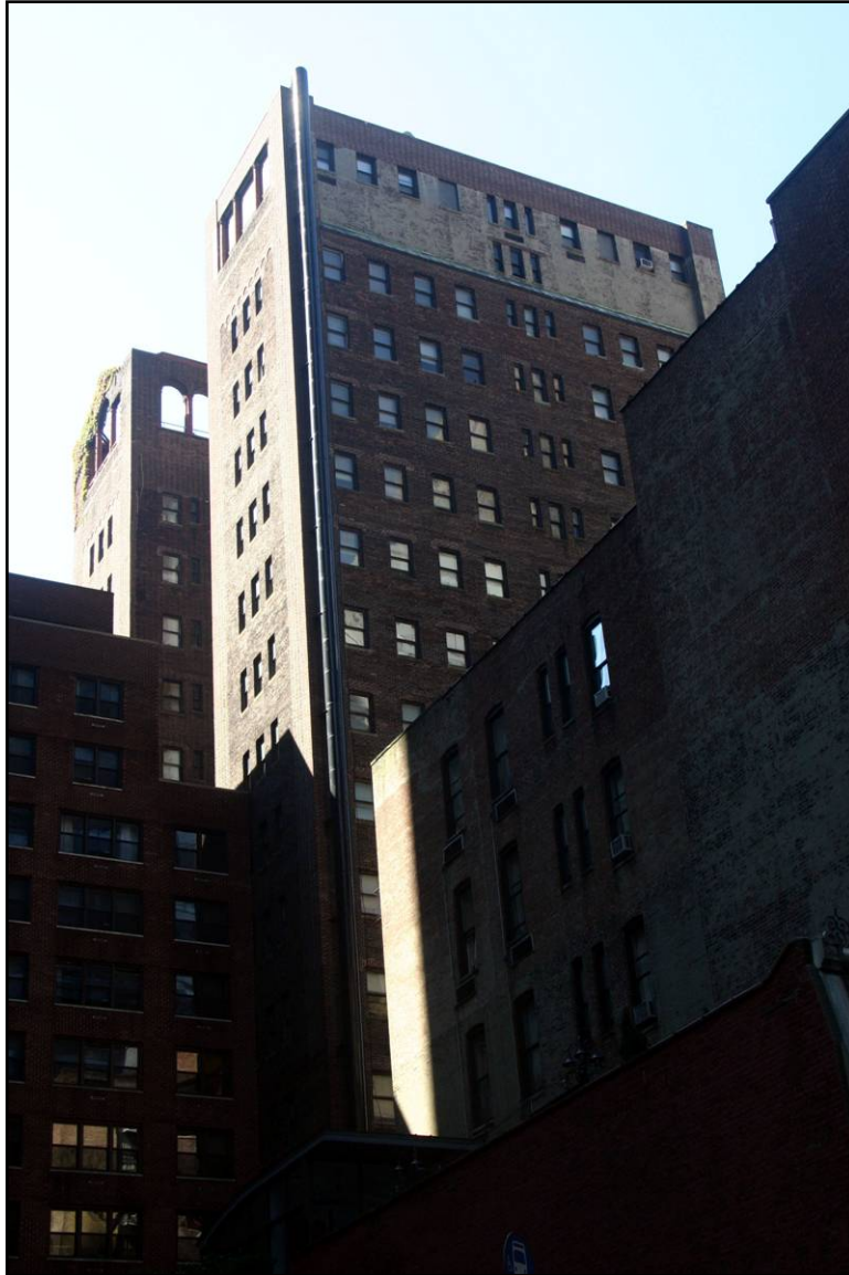
North Elevation Photo by: Carl Forster
