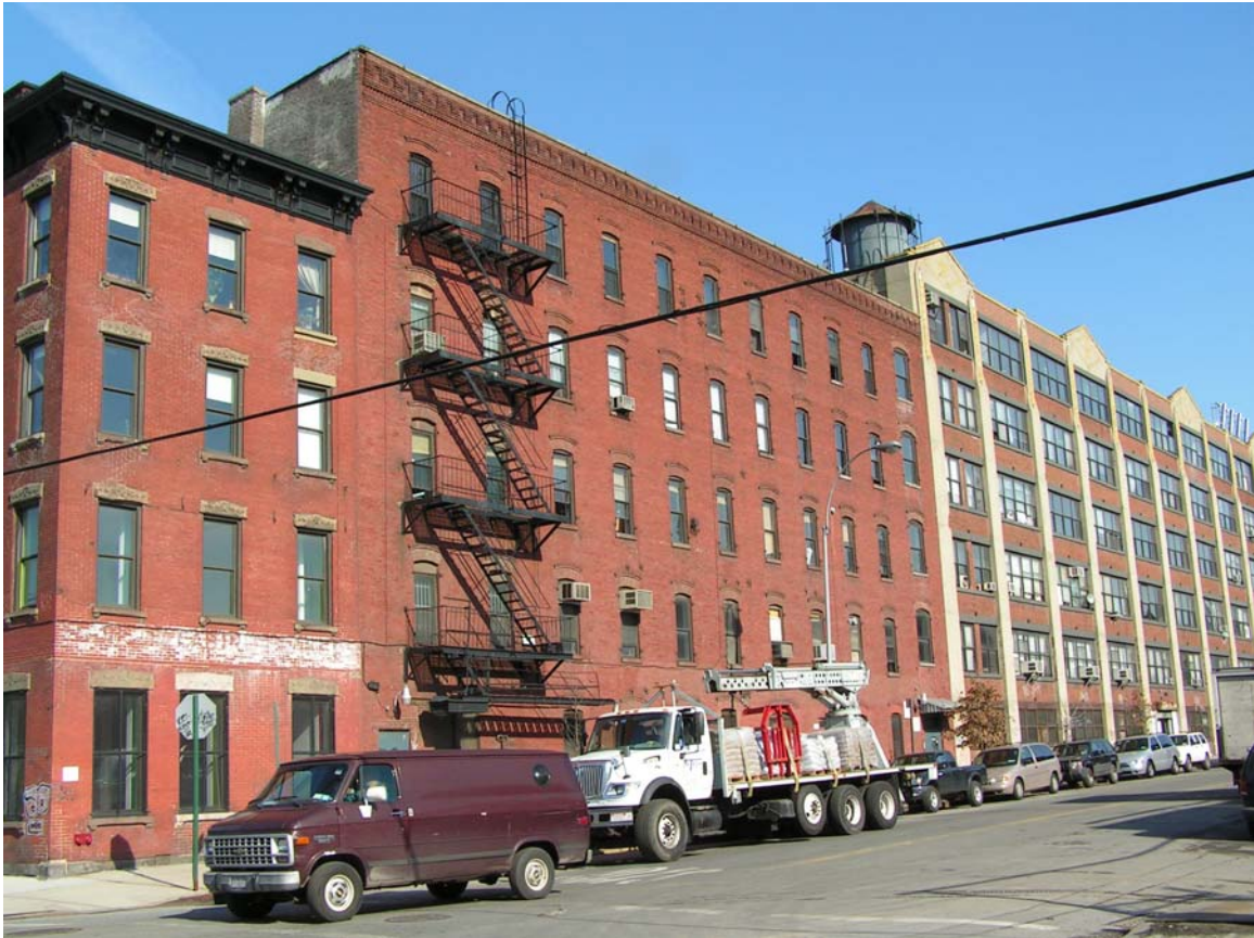
39 to 45 Greenpoint Avenue (at center of view)
