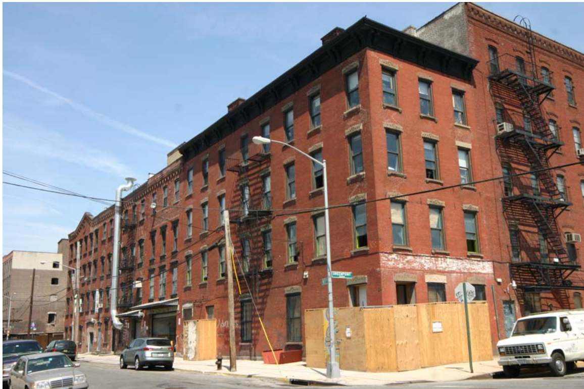
37 Greenpoint Avenue (at the corner)
