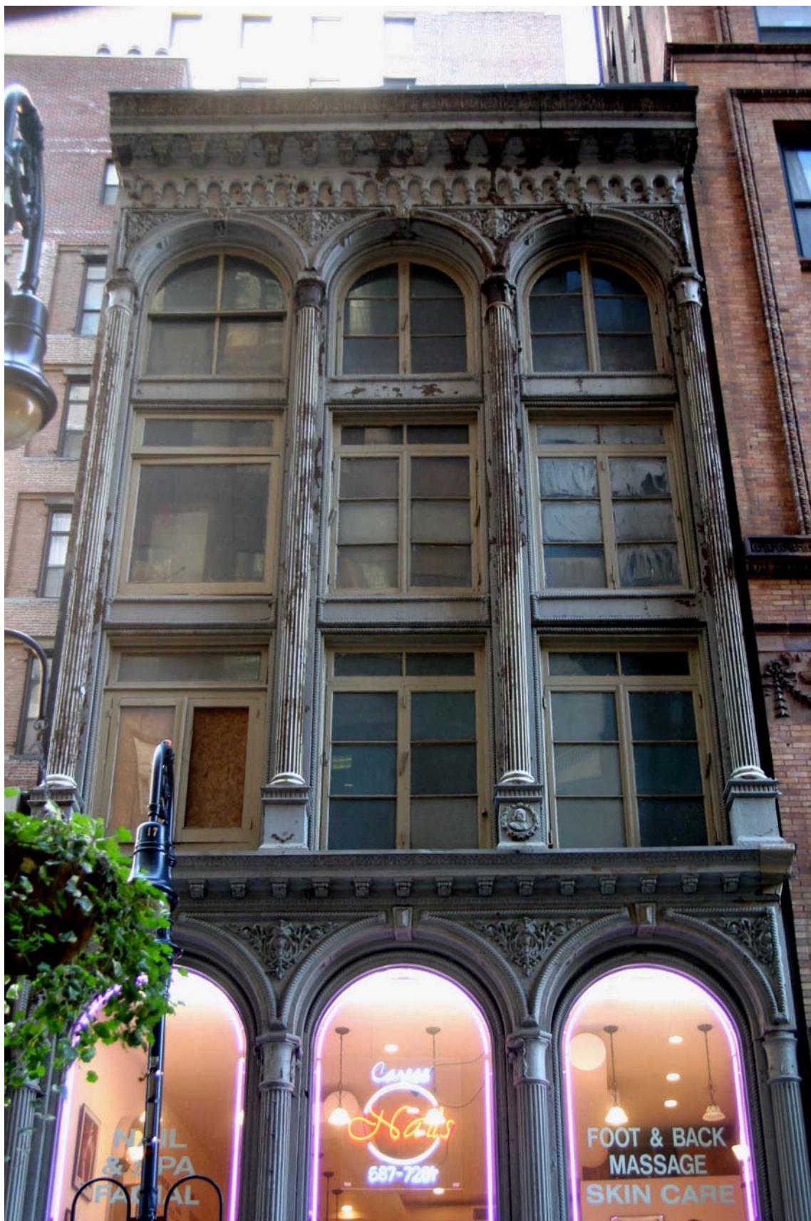
63 Nassau Street Building , Manhattan
