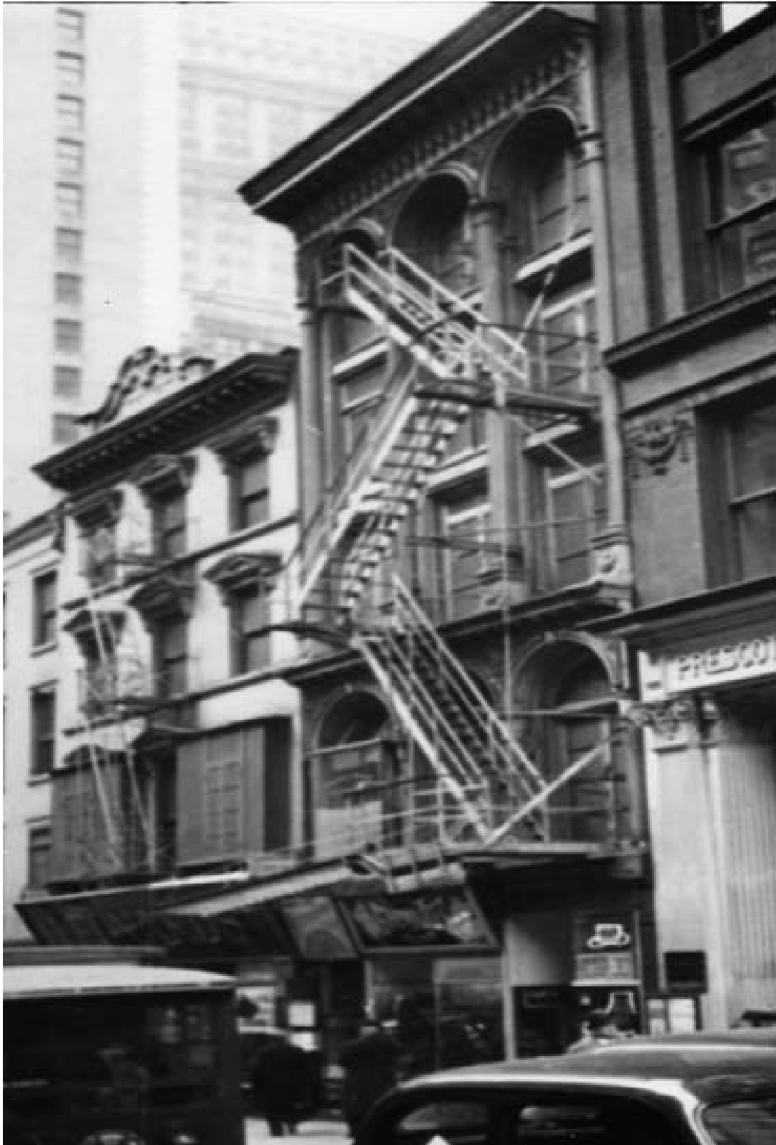
63 Nassau Street Building , Manhattan
