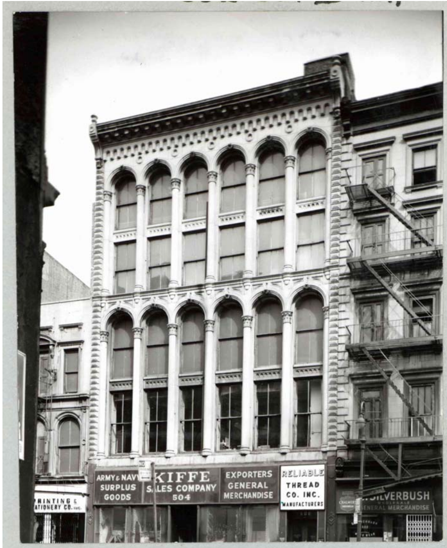
502-504 Broadway (1860, John Kellum & Son), masonry façade
