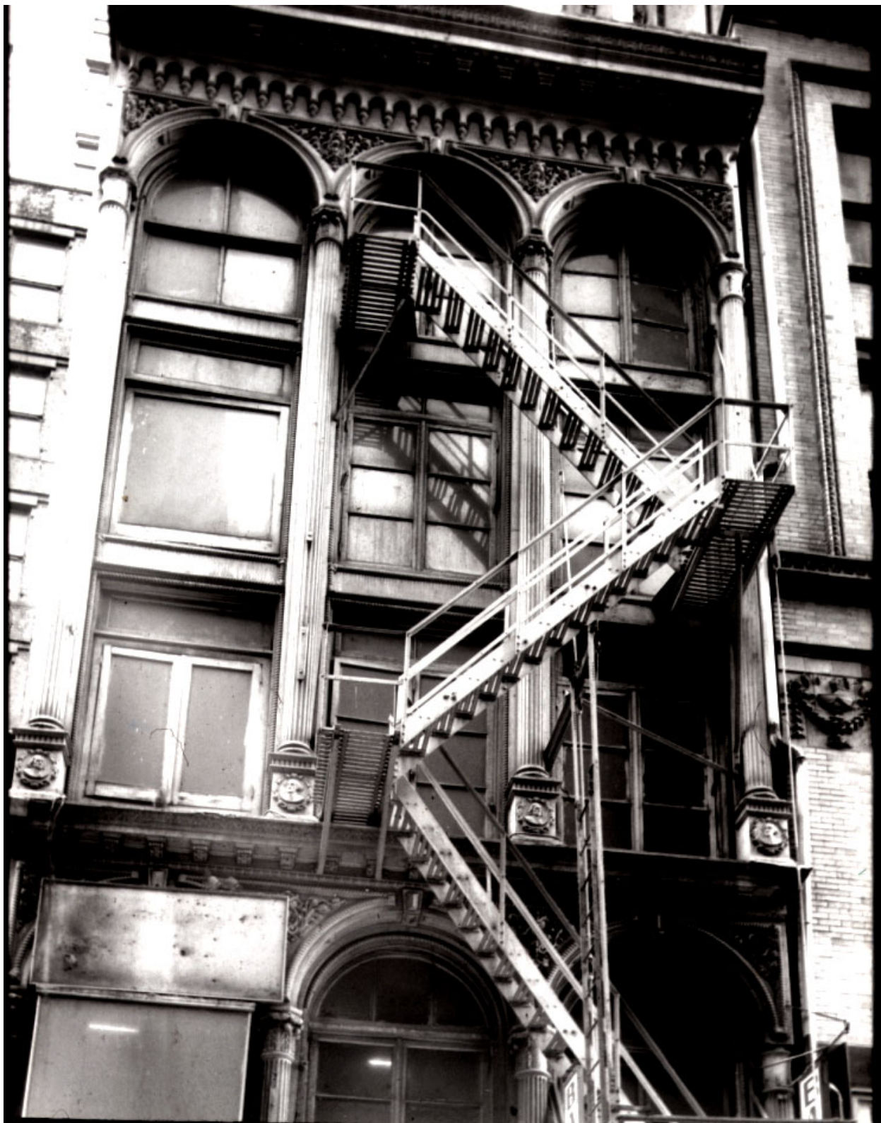
63 Nassau Street Building , Manhattan
