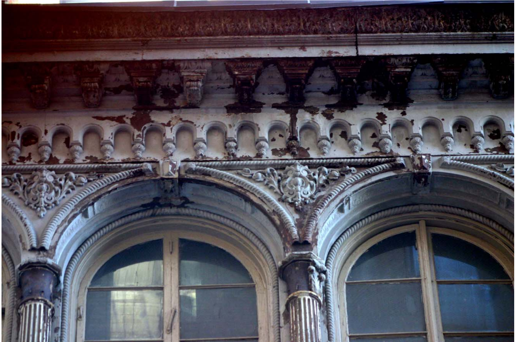
63 Nassau Street Building, cornice
