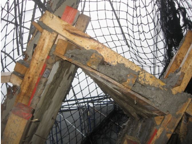
Photo 17 Beam Form (Upside-down)
