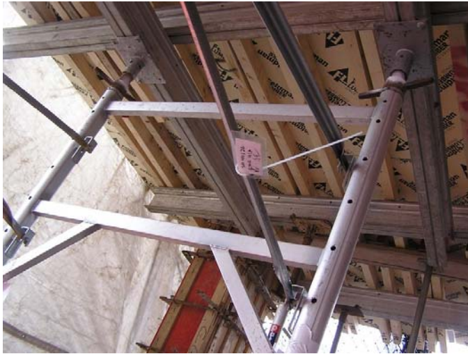
Photo 14 Stringer Supporting Stringer
