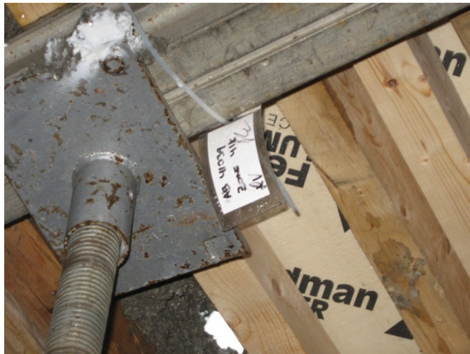
Photo 13 Stringer Set Eccentric on Head Does Not Follow Patent Instructions
