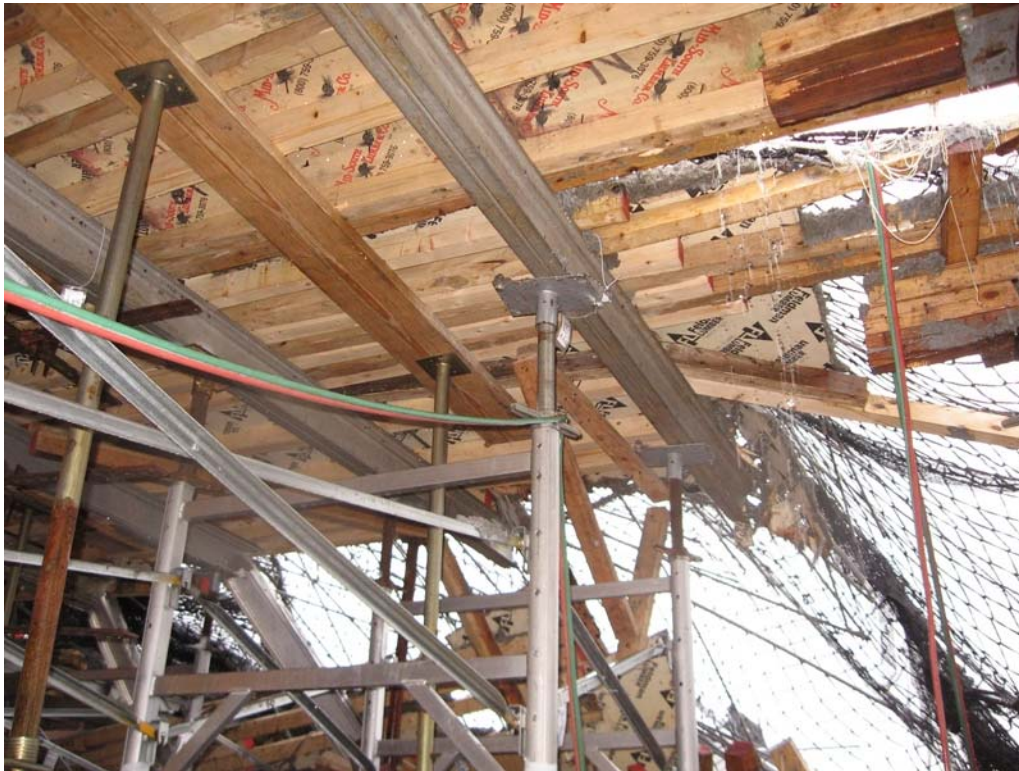
Photo 20 Eccentric Stringer Position on Head
