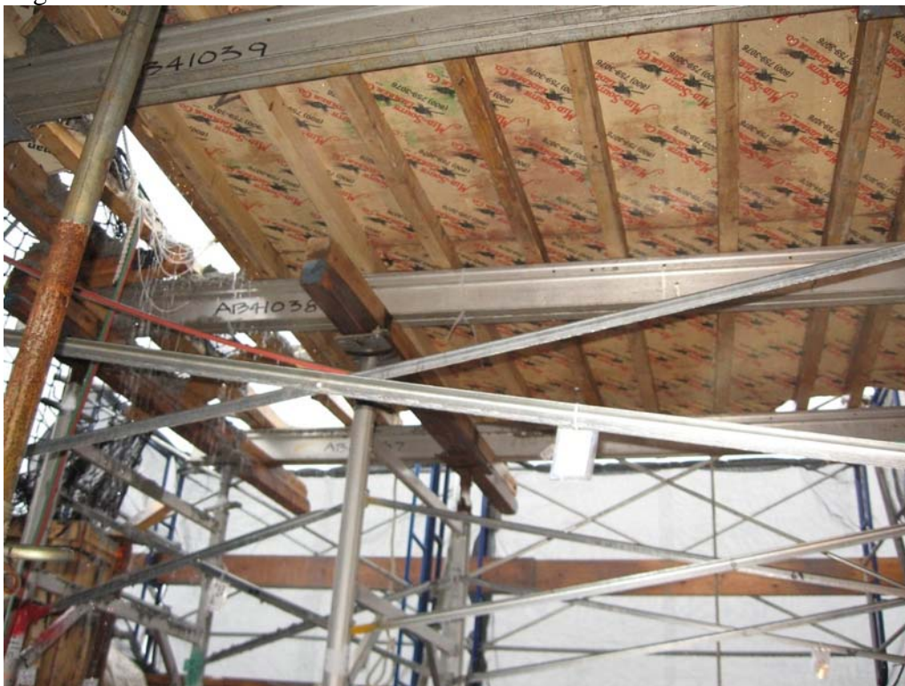
Photo 22 Shoring at the East Side.
