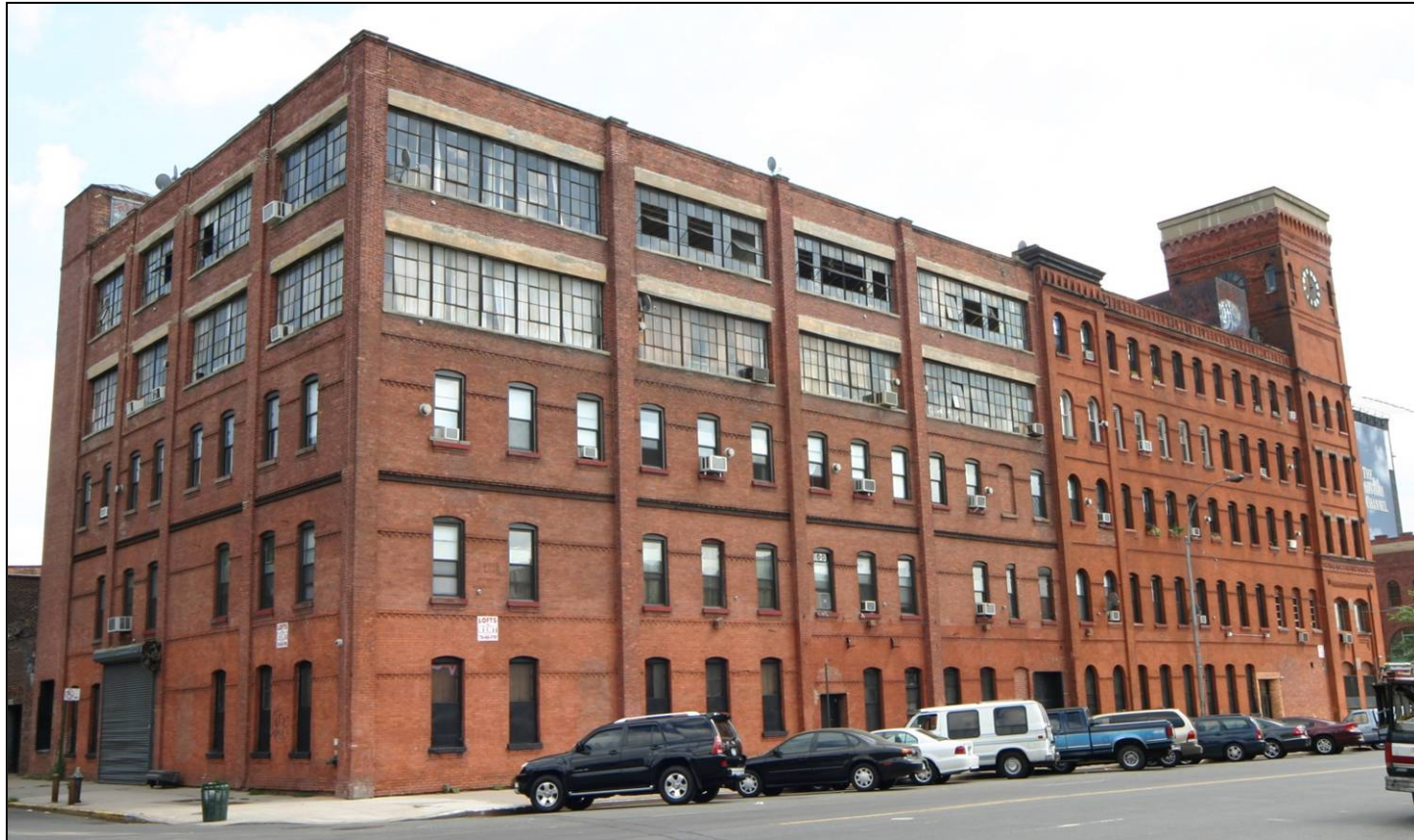
Estey Piano Company Factory, 134 th Street, or north (left) and Lincoln Avenue (center and right) facades. Photo: Carl Forster
