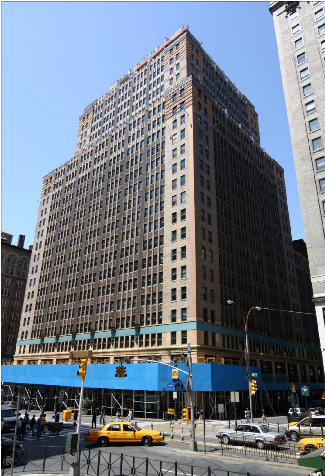
2 PARK AVENUE BUILDING , 2 Park Avenue Manhattan
