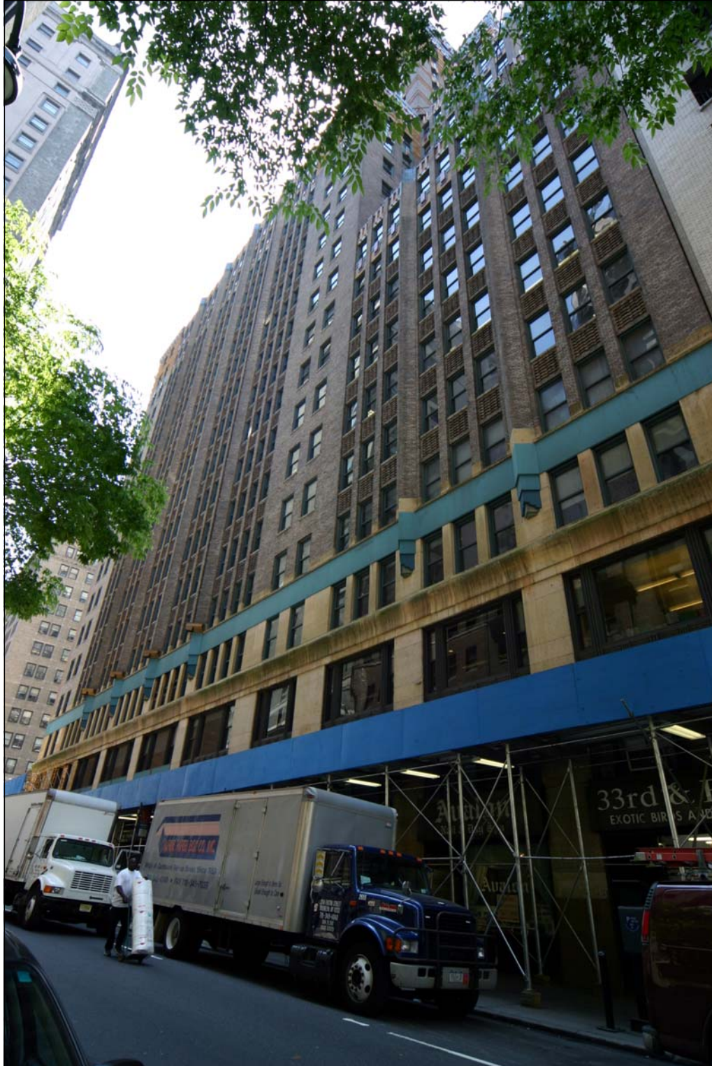
2 PARK AVENUE BUILDING 33rd Street Façade Photo: Carl Forster
