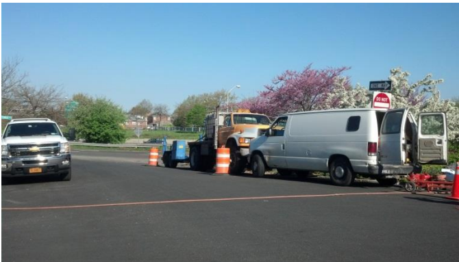
150 th Avenue and 126 th Street, Pre-Construction Work
