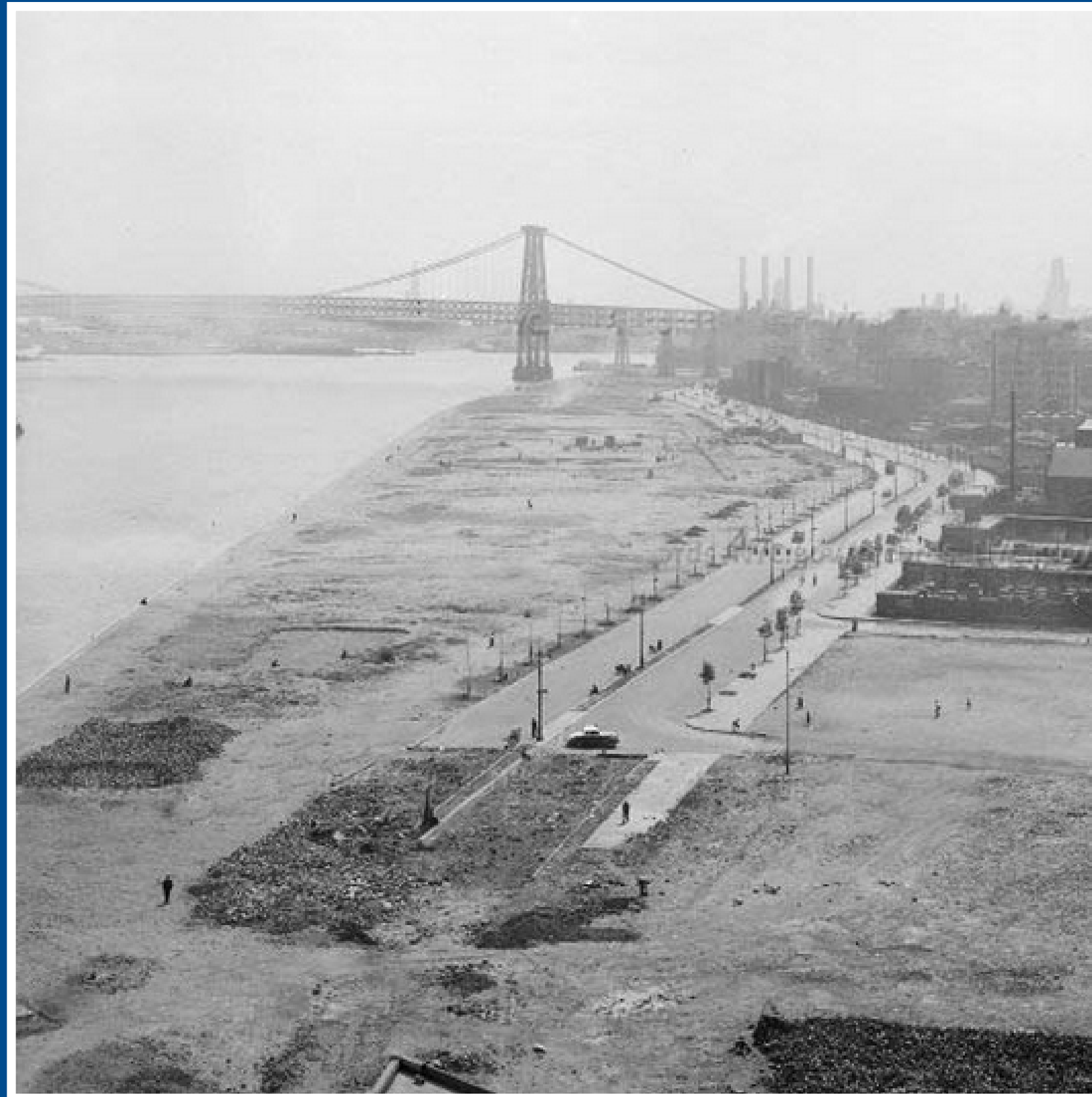
EAST RIVER PARK AND FDR UNDER CONSTRUCTION
