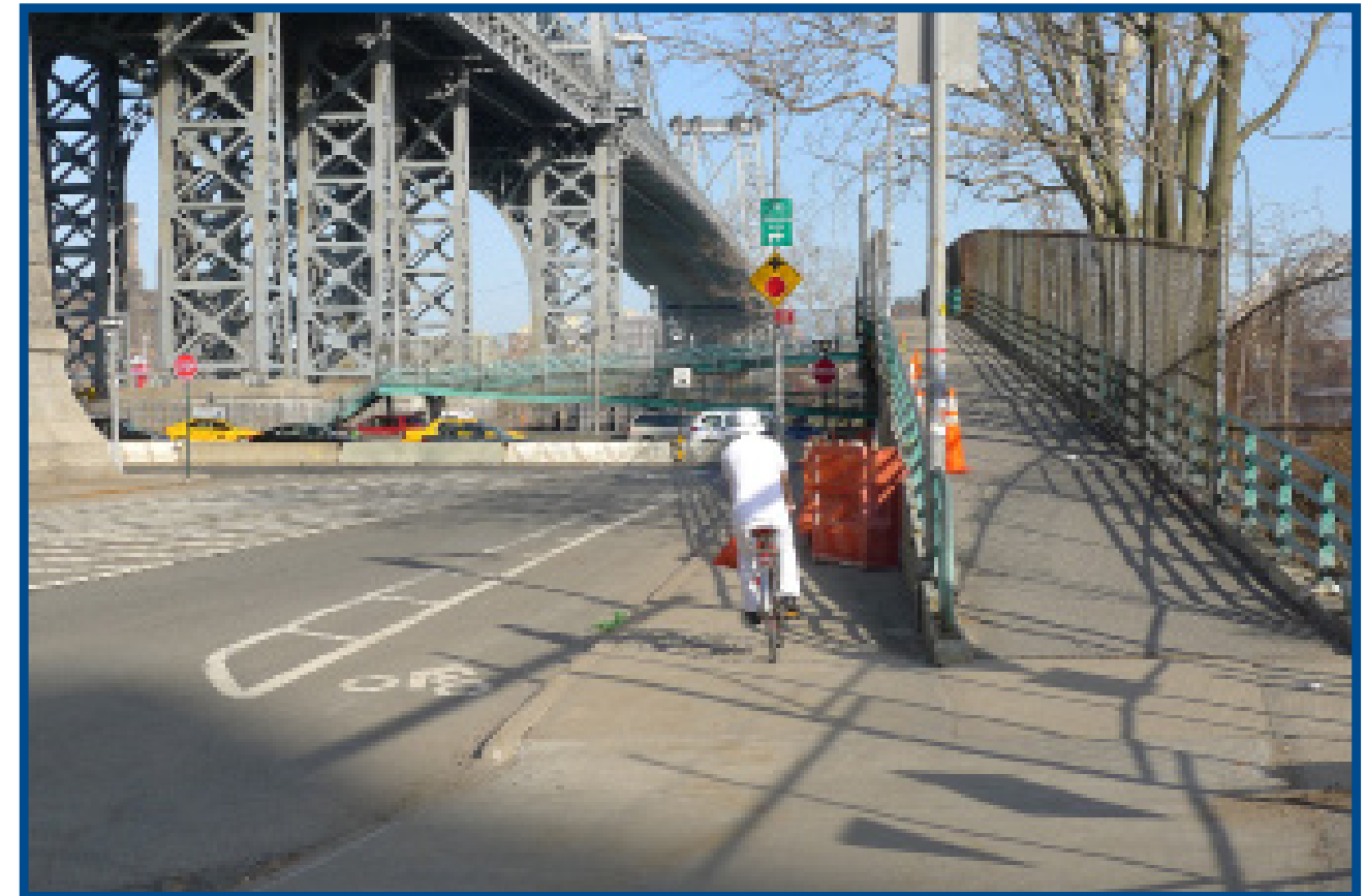
DELANCEY ST. BRIDGE ACCESS POINT
