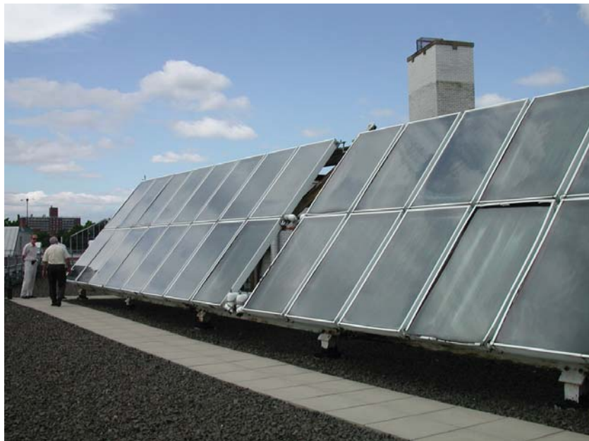
Solar Hot Water Collectors at Bronx High School of Science
