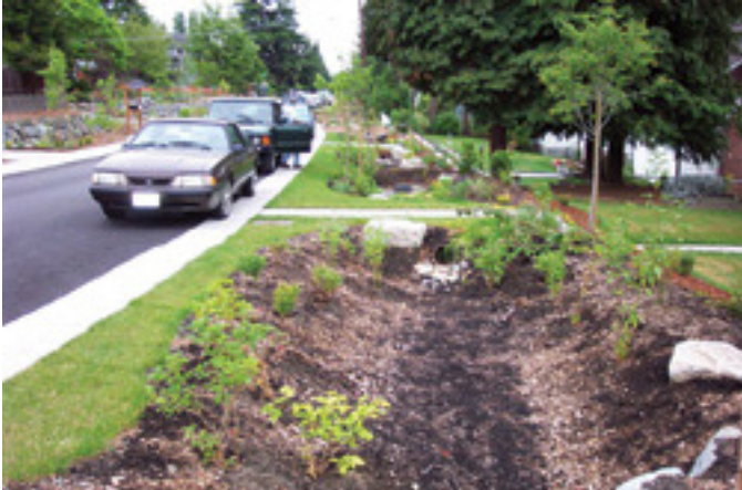
Narrow streets, bordered by beds of dense planting, allow for minimized run-off and natural infiltration. The Street Edge Alternative project (top, left and right) served as a pilot for these approaches, which were then applied when building the 15-block Broadview Green Grid neighborhood (below, left and right).
