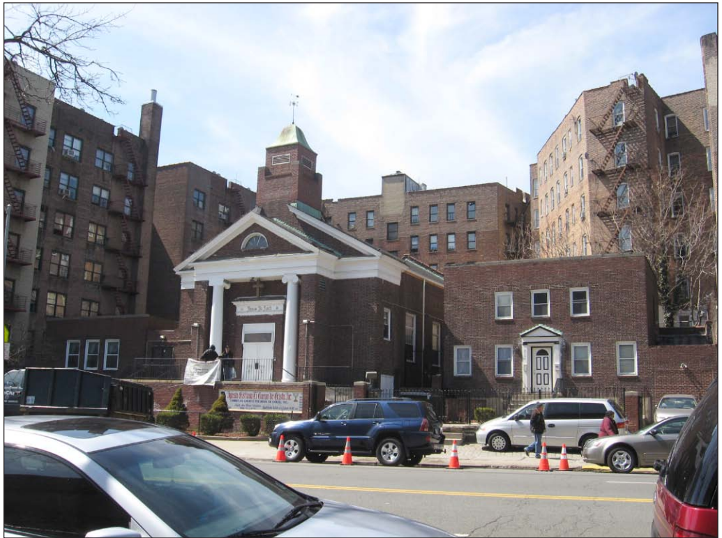
Fordham Manor Reformed Church—2711 Reservoir Avenue 12
