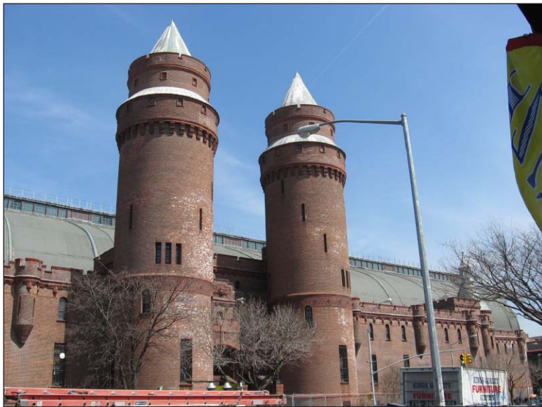
Kingsbridge Armory—View northeast on West Kingsbridge Road to the Armory's south facade 3
