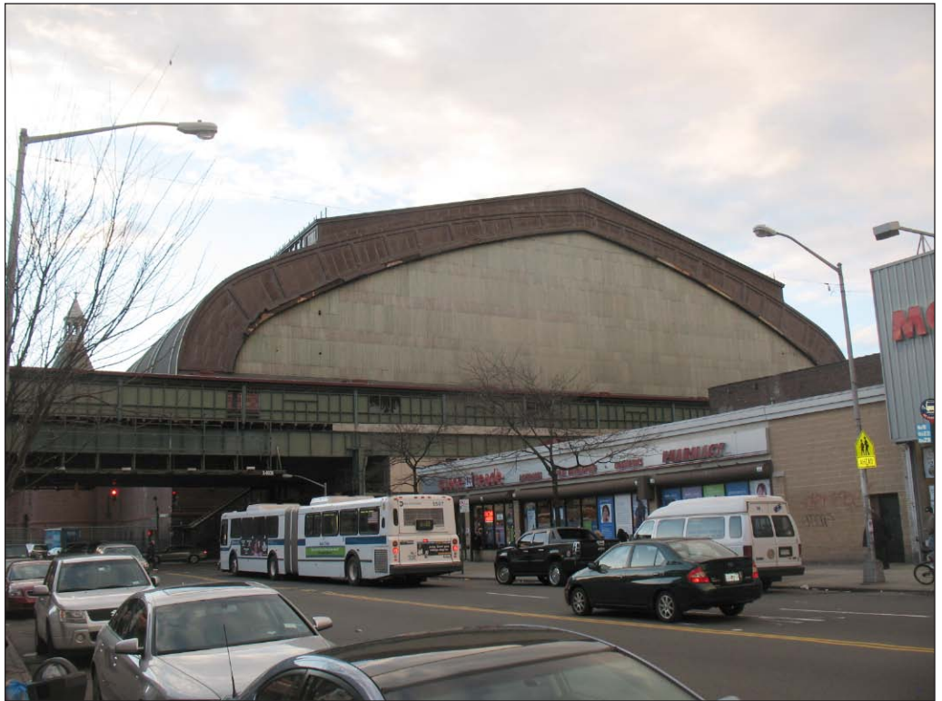
Kingsbridge Armory—View northwest on East Kingsbridge Road to the Armory's east facade 8
