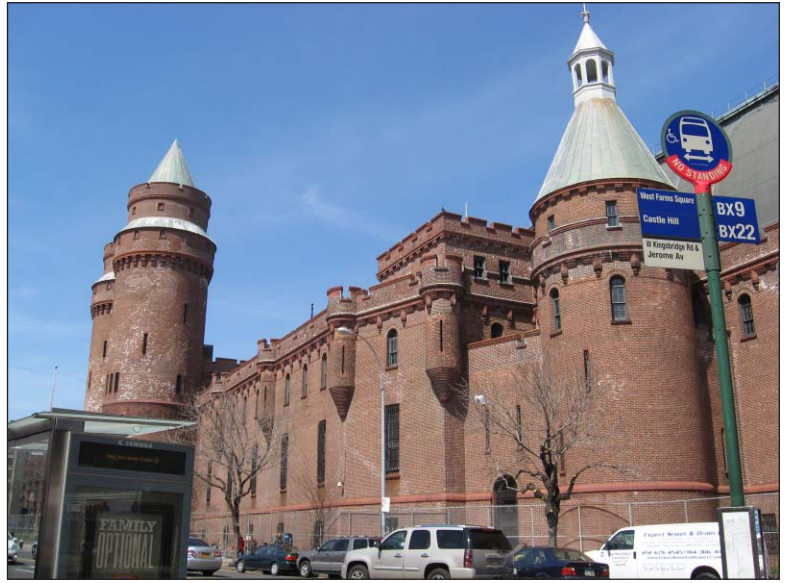
Kingsbridge Armory—View northwest on West Kingsbridge Road to the Armory's south facade 2
