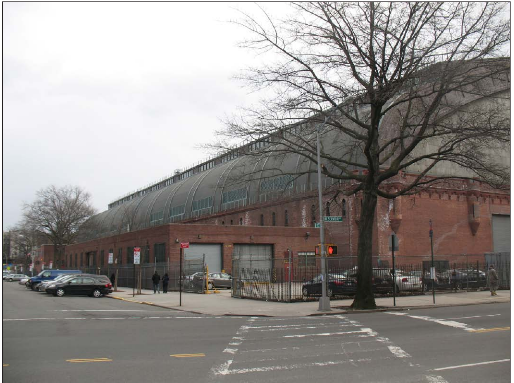
Kingsbridge Armory—View southeast on Reservoir Avenue to the Armory's north facade 6
