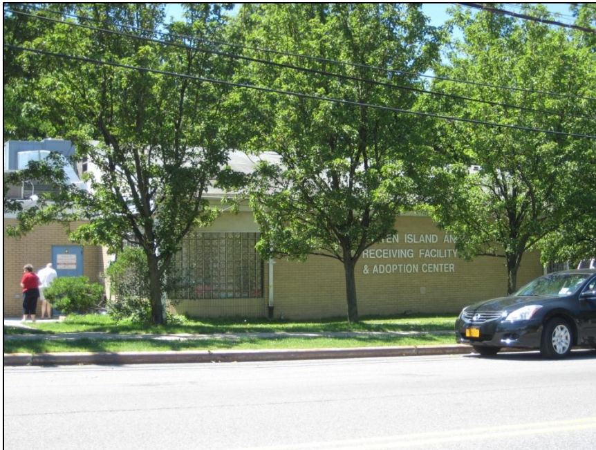
View of a one-story community facility/institutional building located on the south side of Veterans Road West.
