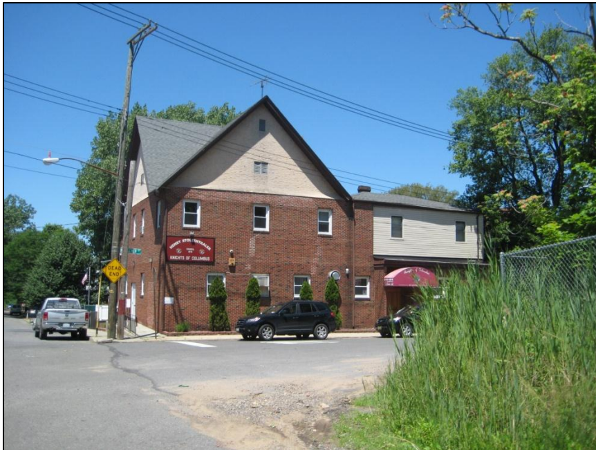
View of a converted two-story community facility building at the northwest corner of Androvette and Kreisler Streets.
