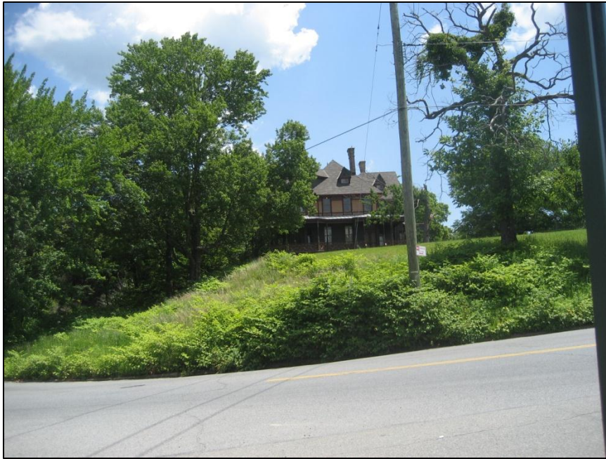
View of the former Kreischer mansion along the east side of Arthur Kill Road at Kreischer Street.
