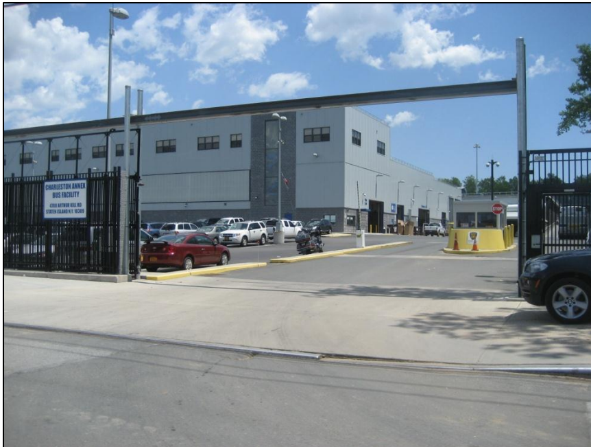
View of the MTA bus depot looking northeast from Arthur Kill Road.
