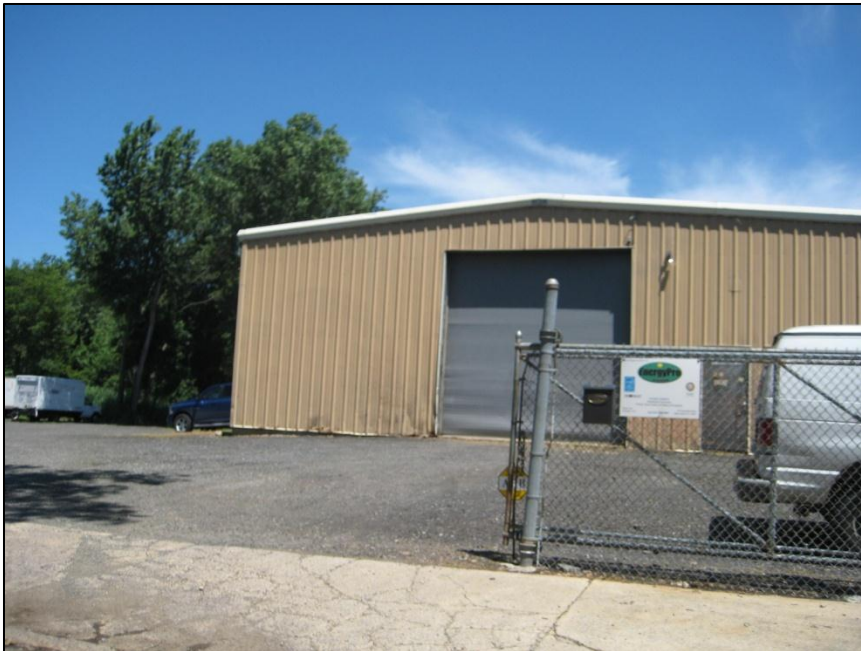
View of a one-story warehouse storage building along the north side of Androvette Street, near the Arthur Kill waterfront.
