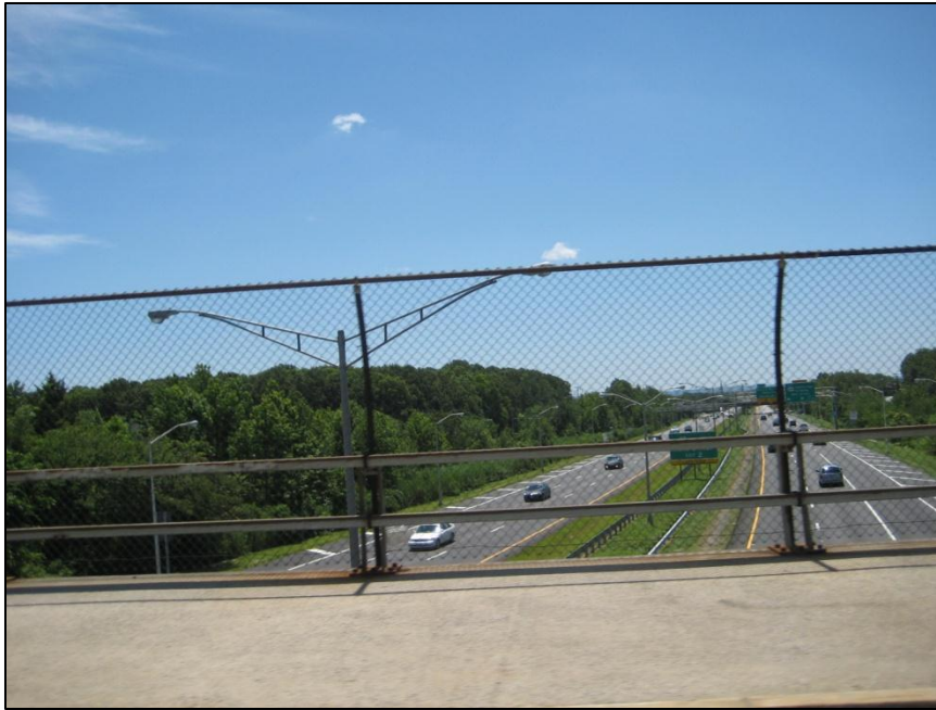
View of the West Shore Expressway from the overpass along Englewood Avenue.
