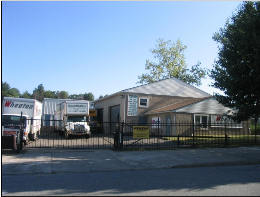
View of an existing one-story industrial building along the north side of Veterans Road West, south of the Project Area.
