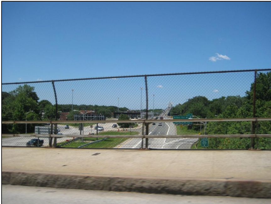
View looking west towards the Outerbridge Crossing.
