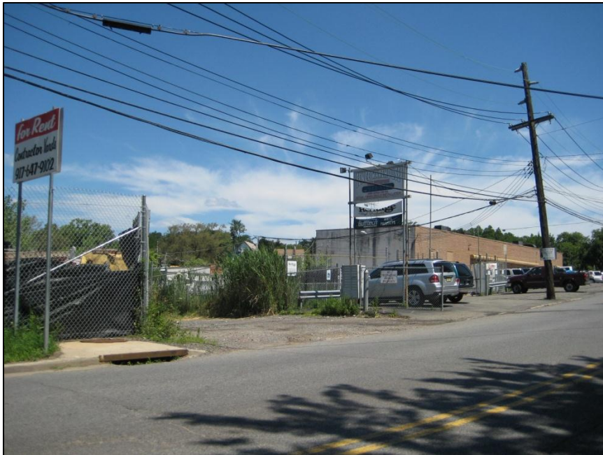
View of one-story commercial buildings along the west side of Arthur Kill Road, across from Englewood Avenue.
