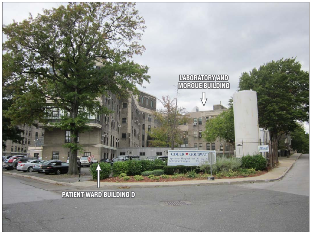
View northeast to the Laboratory and Morgue Building's east facade, with Patient Ward Building D in the foreground
