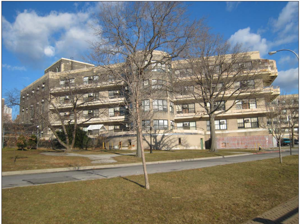
Patient Ward A—View northwest to the east wing's south facade 4
