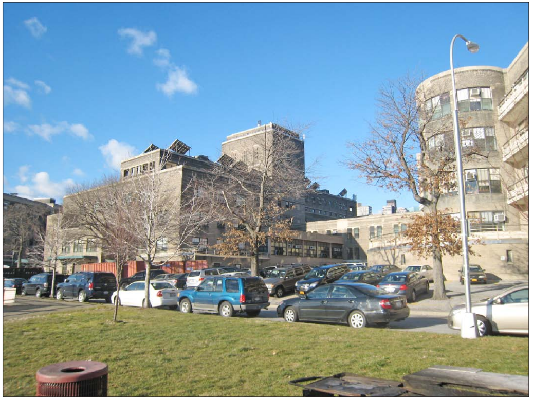
View west to the Administration Building and Patient Ward Building D 2
