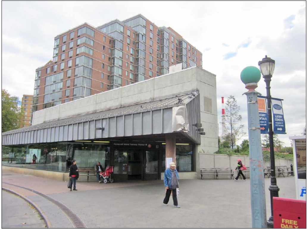
Roosevelt Island Subway Station 33
