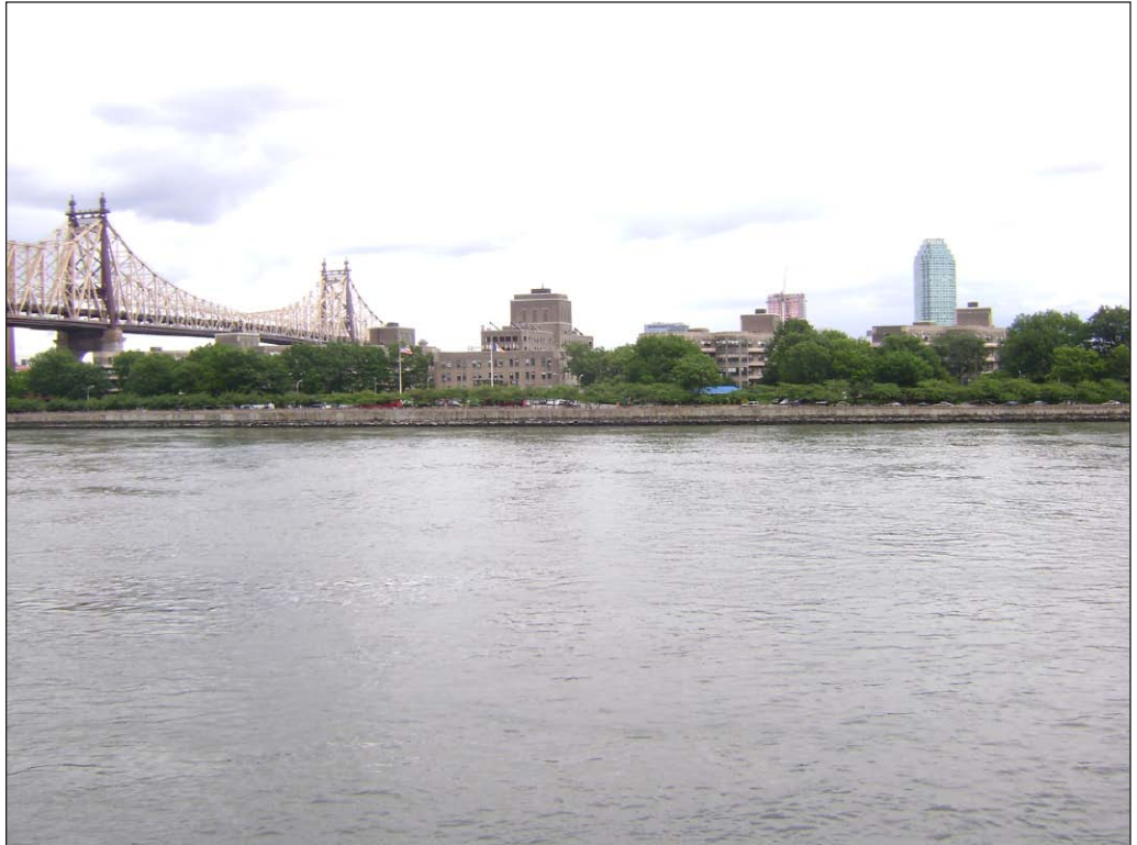
View east to project site from Sutton Place Park 49
