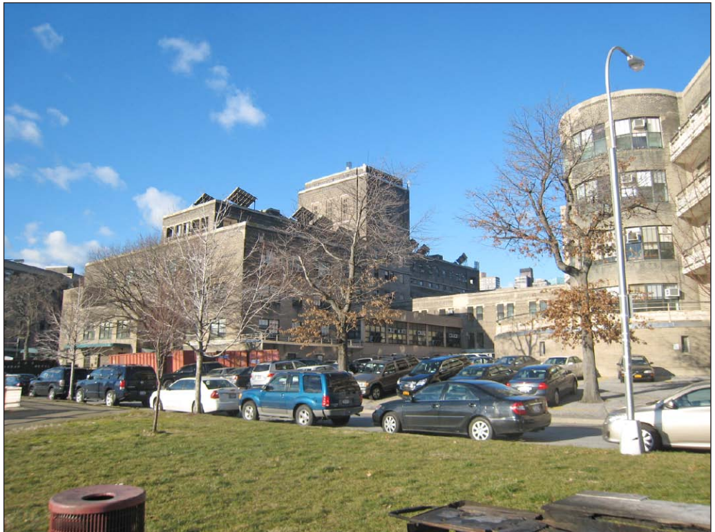
Building E, view of east side 2
