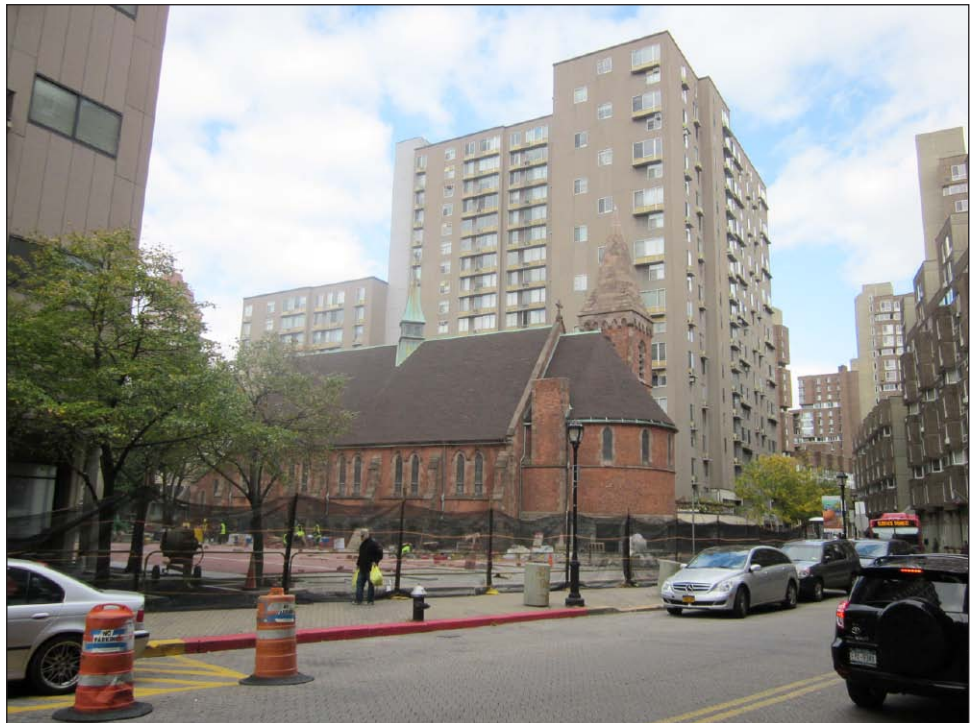
Chapel of the Good Shepherd and Island House in the background 22
