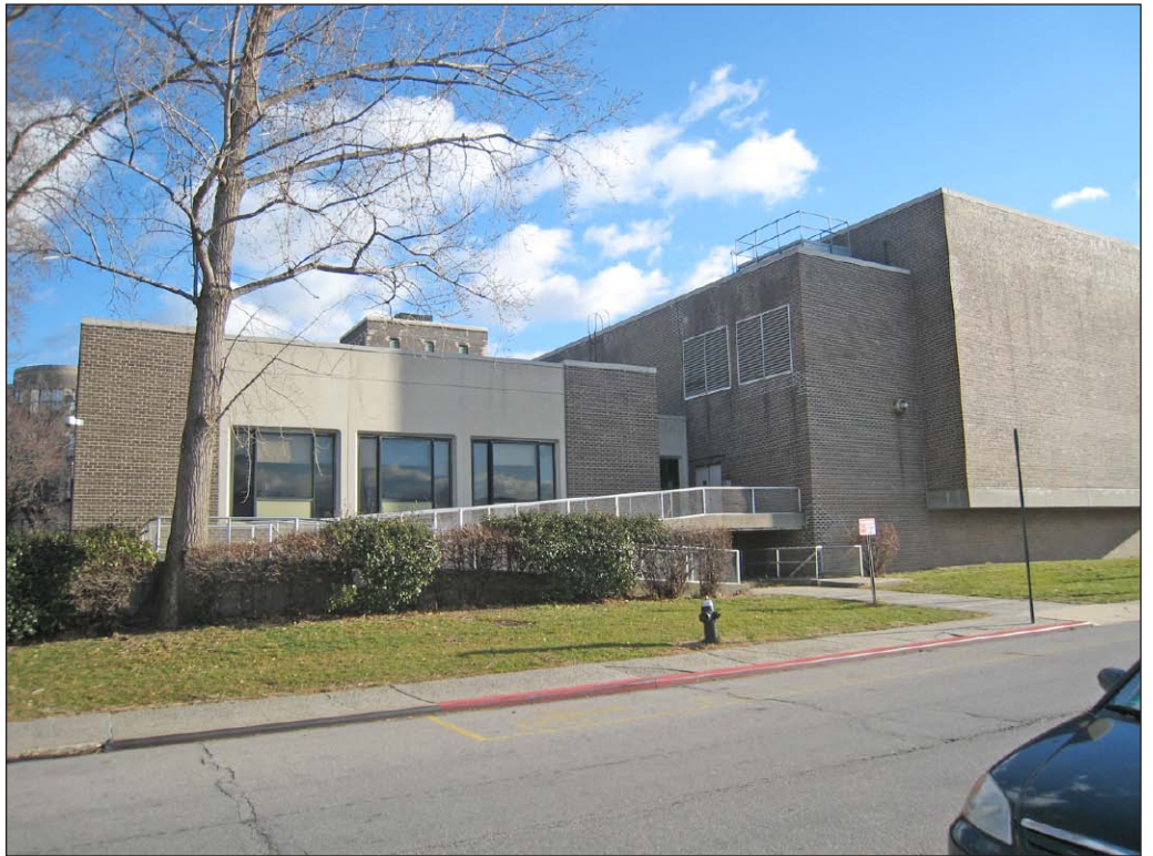
View of southern facade of Building J 6
