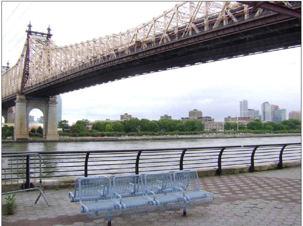
View southeast to project site from Manhattan north of Queensboro Bridge 50
