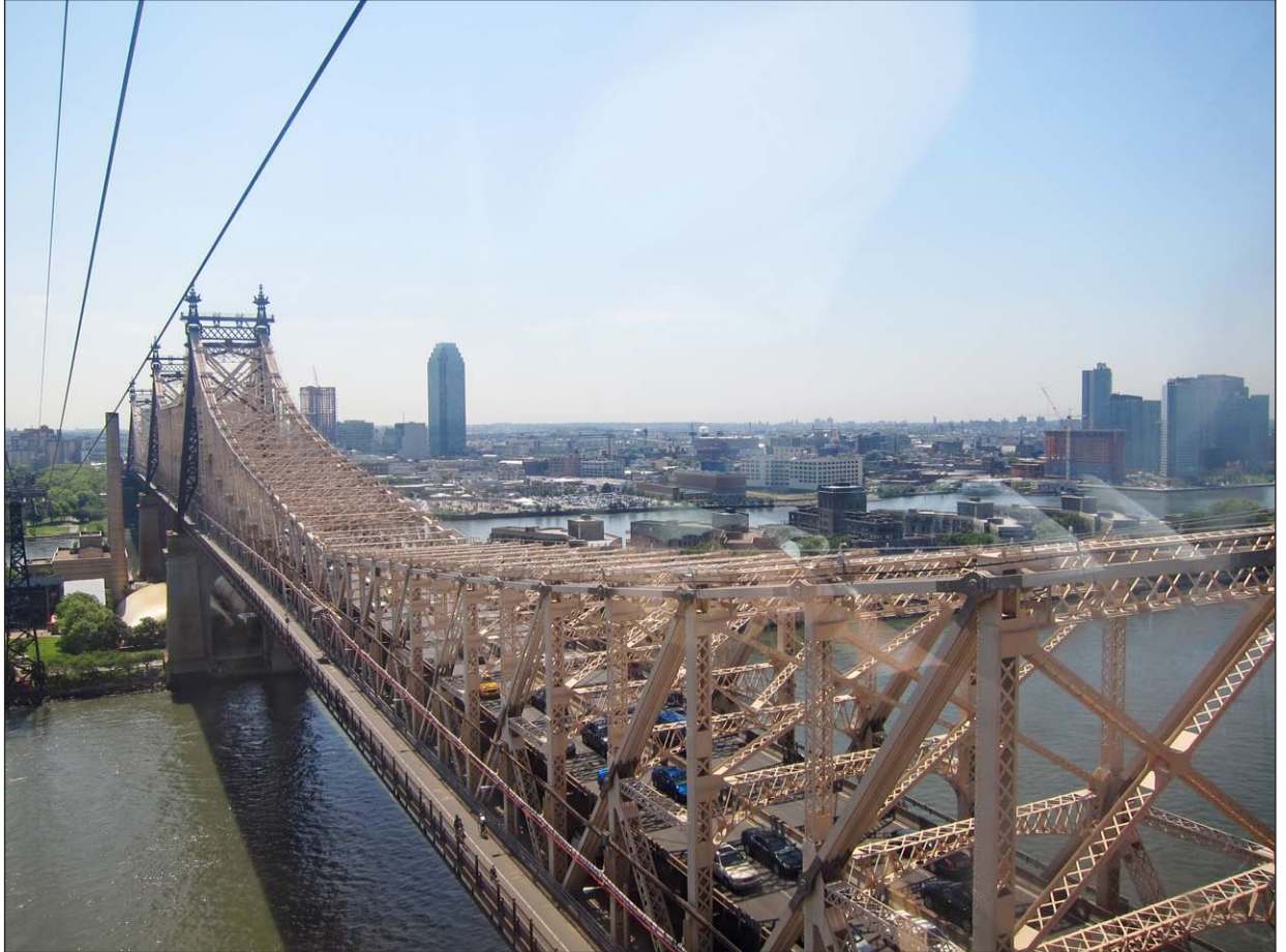
View to project site from Roosevelt Island Tram 53
