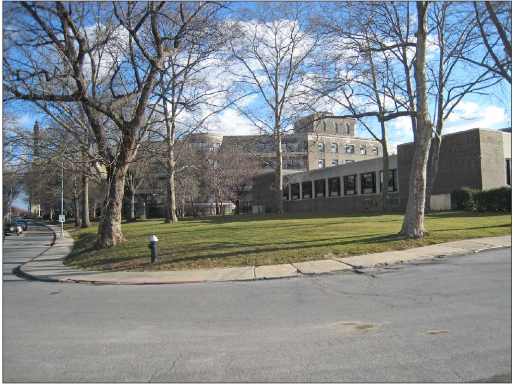
View of western facade of Building J 5
