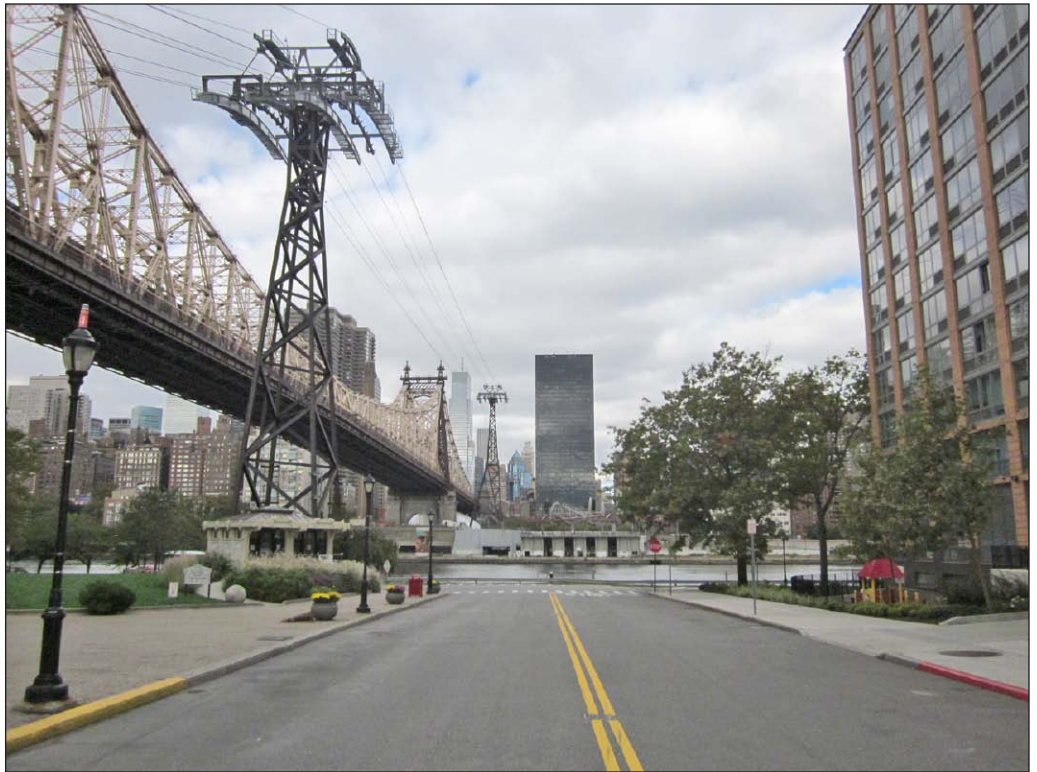
View west along Road 5 16
