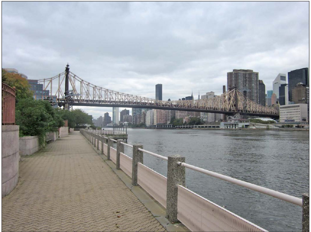
View south along western promenade of Ed Koch-Queensboro Bridge 18
