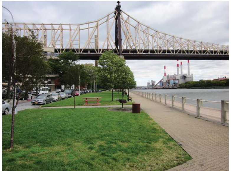
Northern section of eastern promenade looking north
