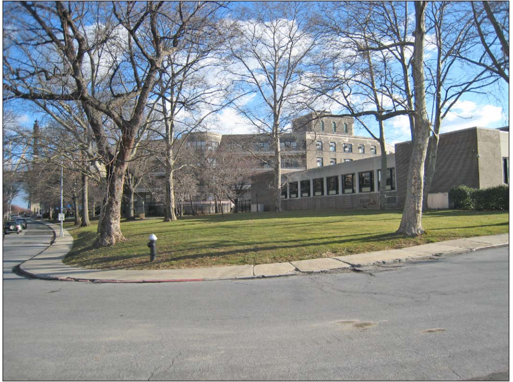
View northeast to the Activities Building/Building J, with Patient Ward Building A in the background 8
