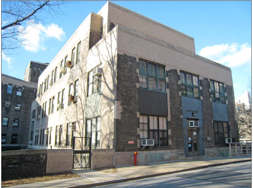
View of northern facade of Building F 7
