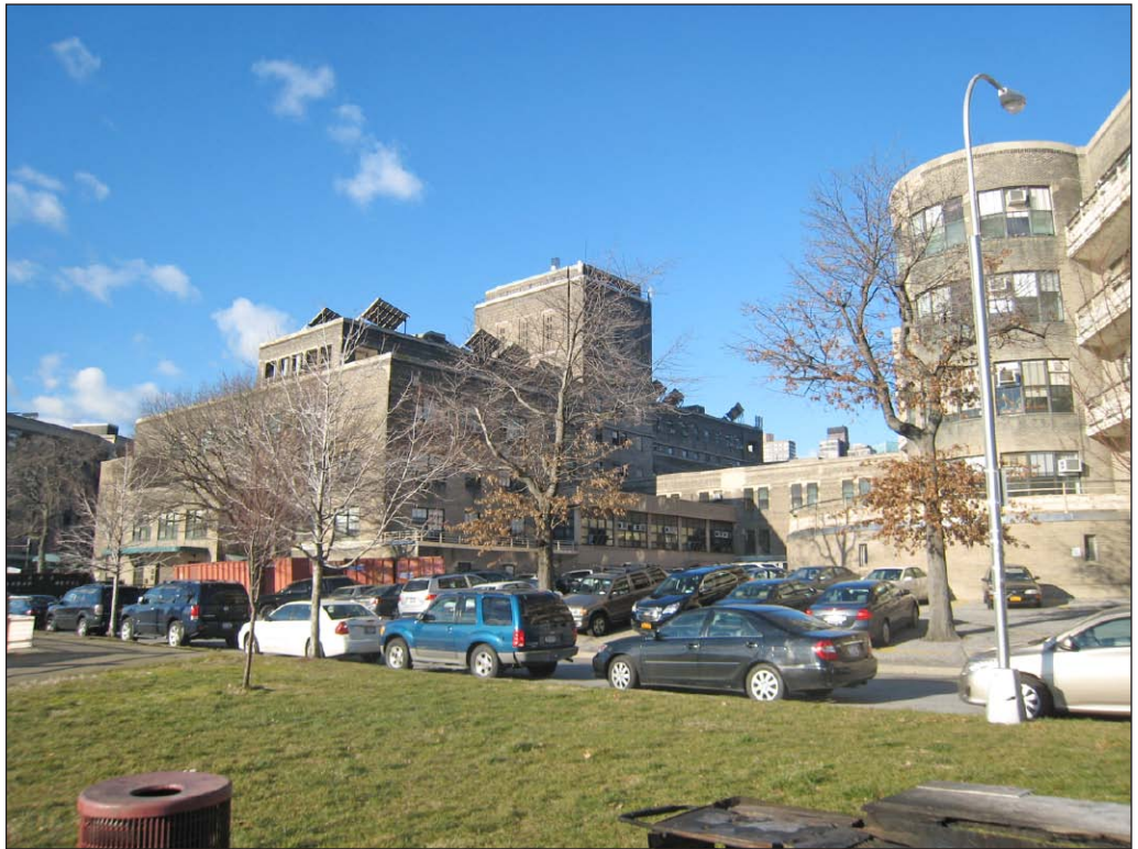
Building E, view of east side 2
