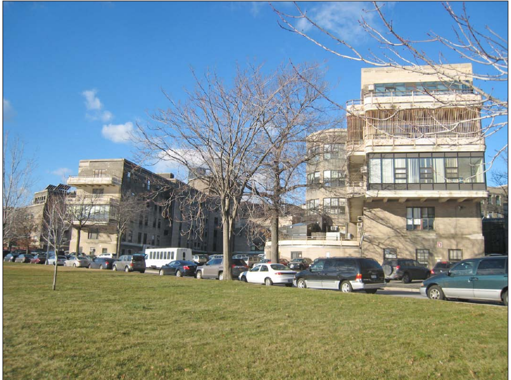
Buildings C and D, view looking southwest 1
