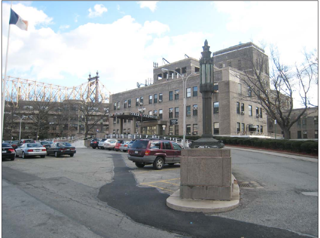
View of ornate lamps flanking main entrance 3
