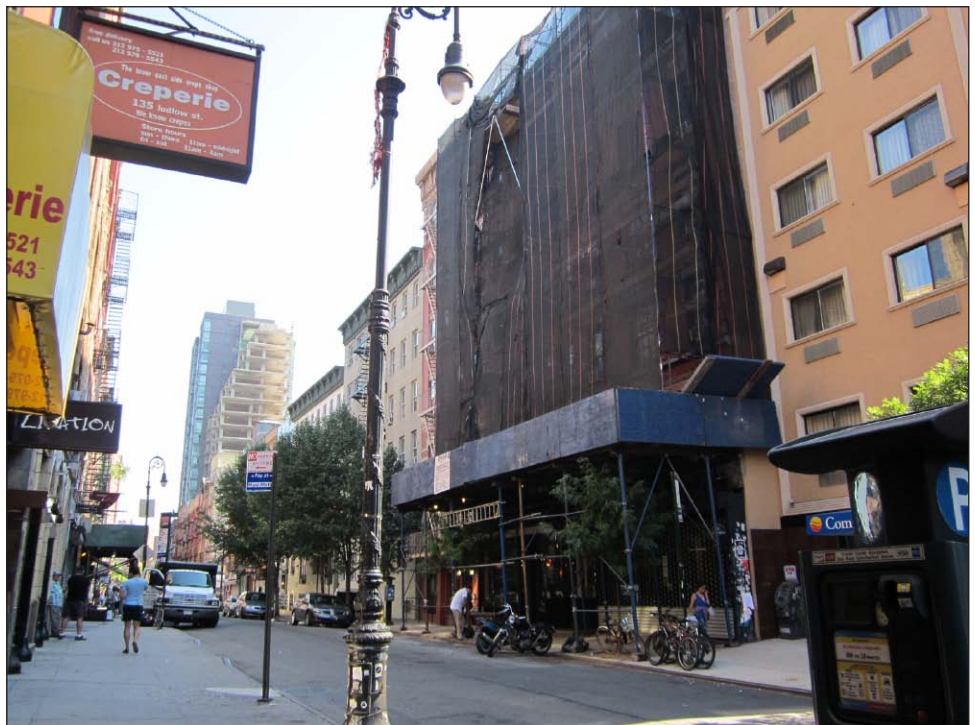
Ludlow Street, view north from Rivington Street 28
