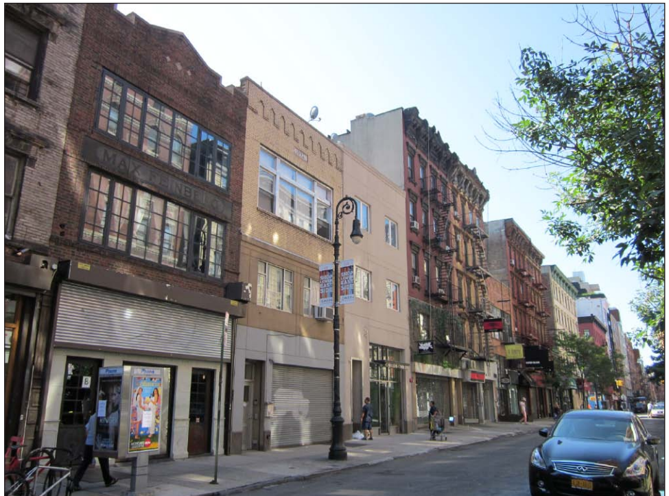
Orchard Street, view south from Broome Street 26
