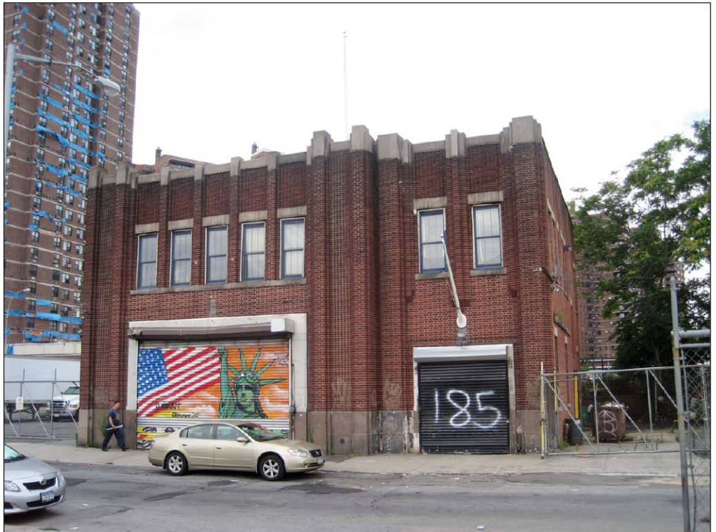
Site 5 – 185 Broome Street (#2) 2
