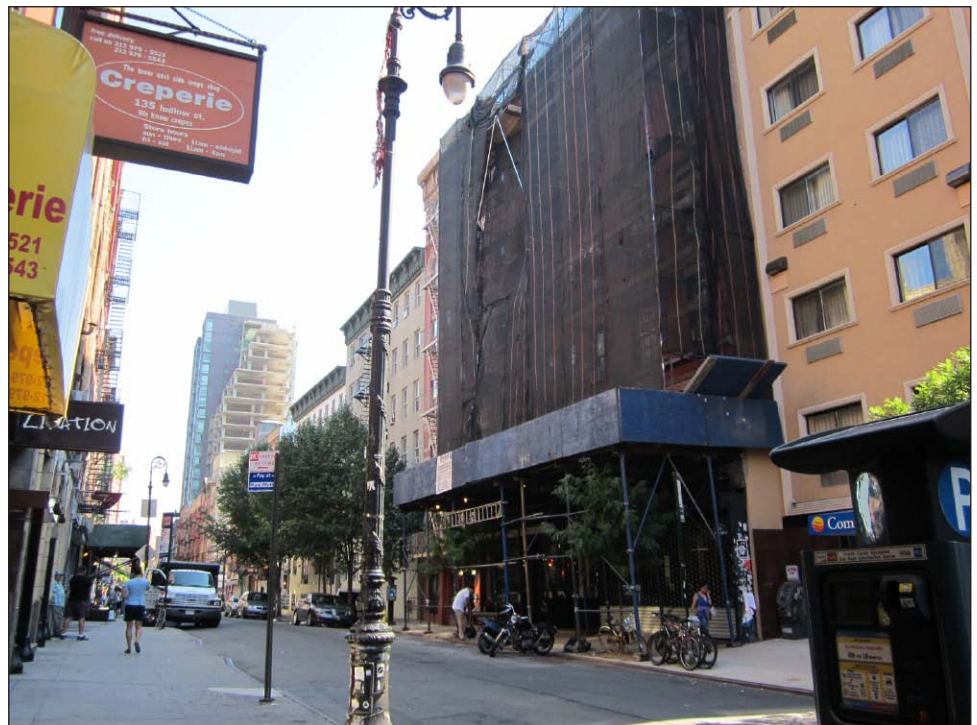
Ludlow Street, view north from Rivington Street 28
