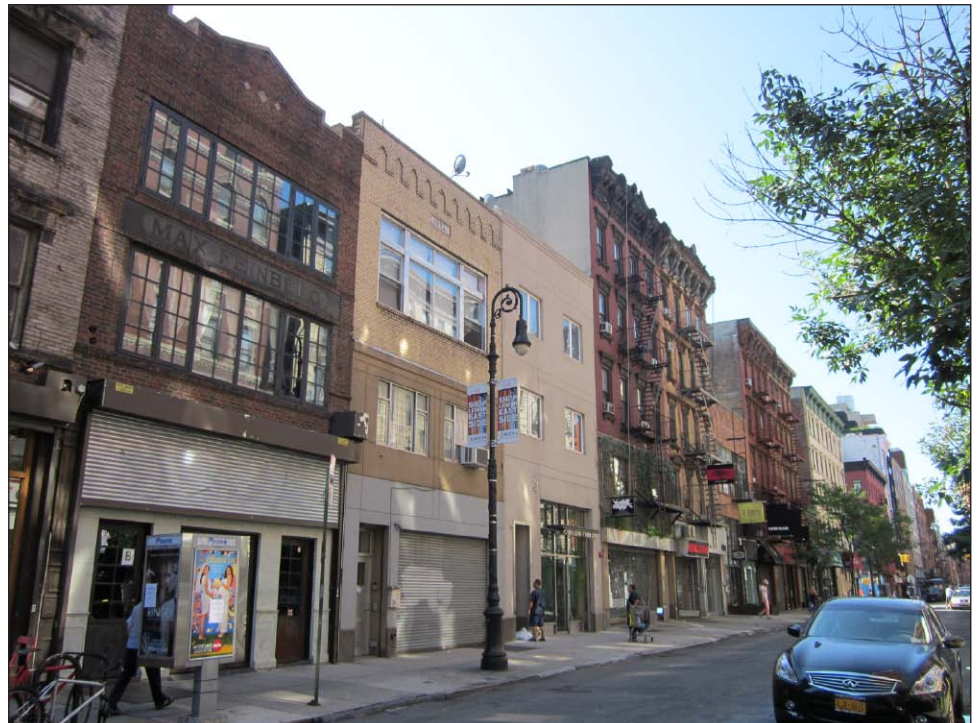
Orchard Street, view south from Broome Street 26
