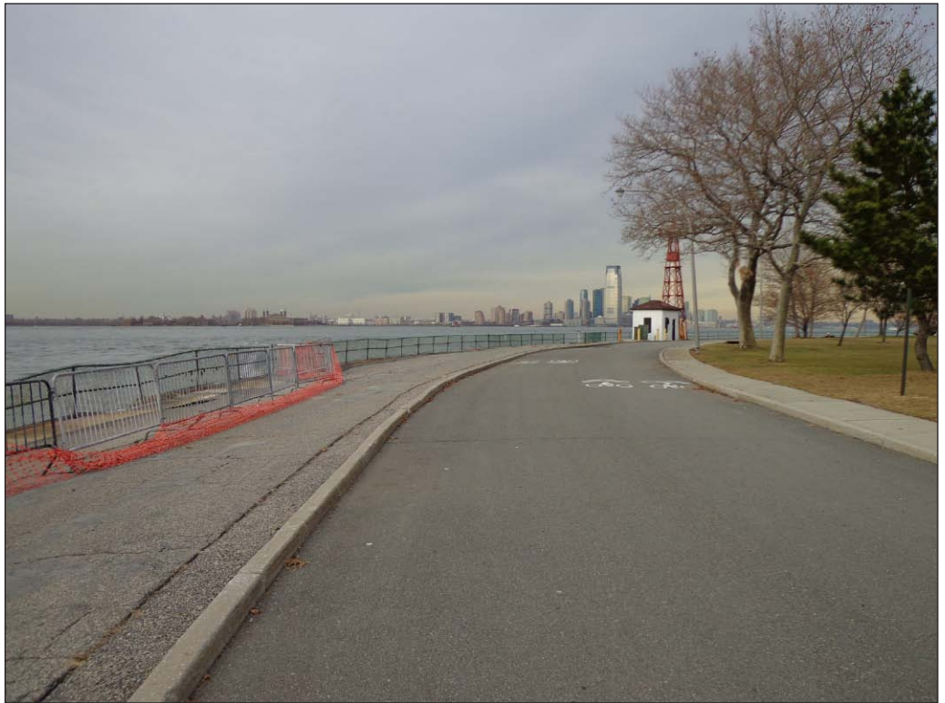
Waterfront esplanade and seawall, at Picnic Point 30
