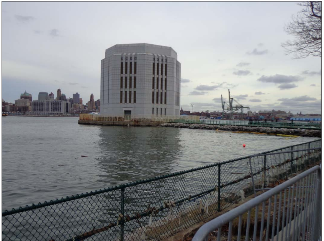
Brooklyn-Battery Tunnel Ventilation Structure 16
