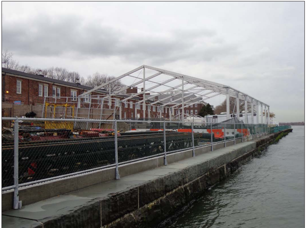
Soissons Concession Site, view west 14
