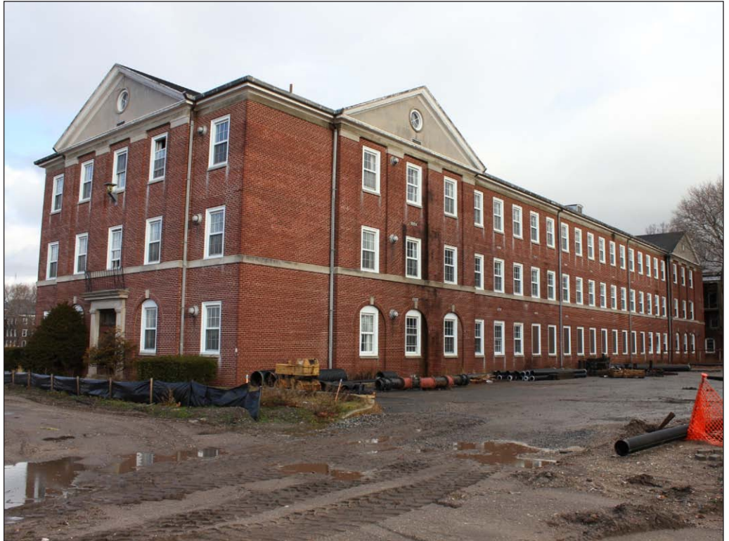
Building 400, Wing O 9
