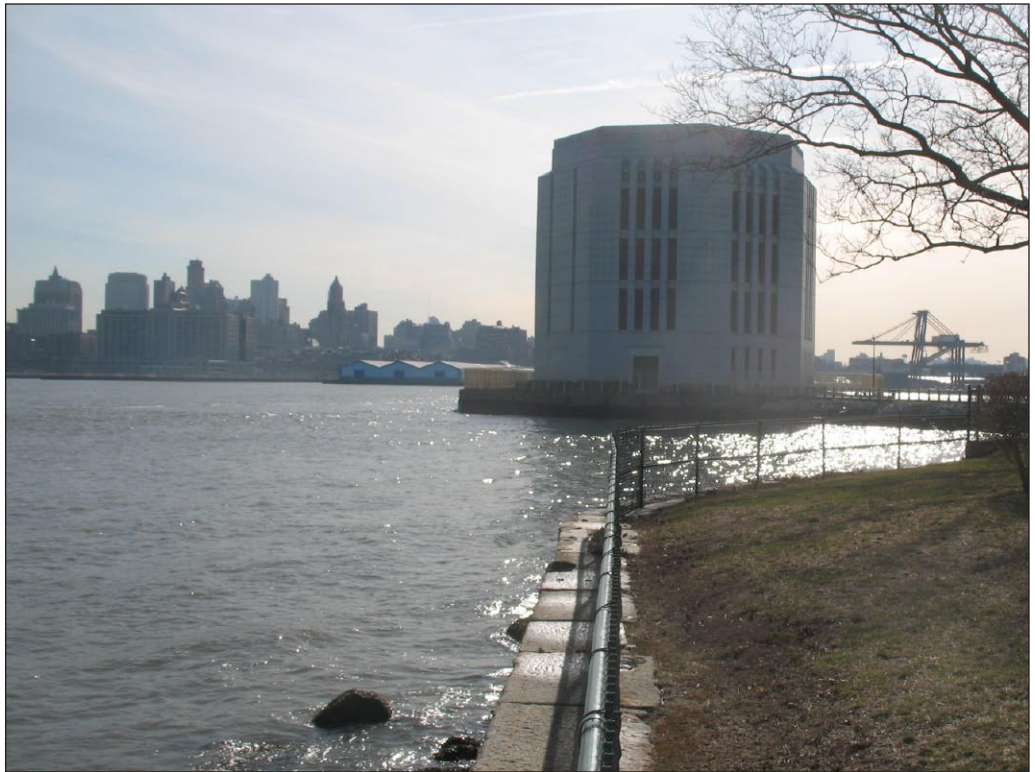
Brooklyn-Battery Tunnel Ventilation Structure 12
