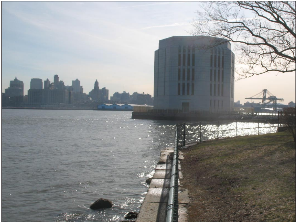
Brooklyn-Battery Tunnel Ventilation Structure 12
