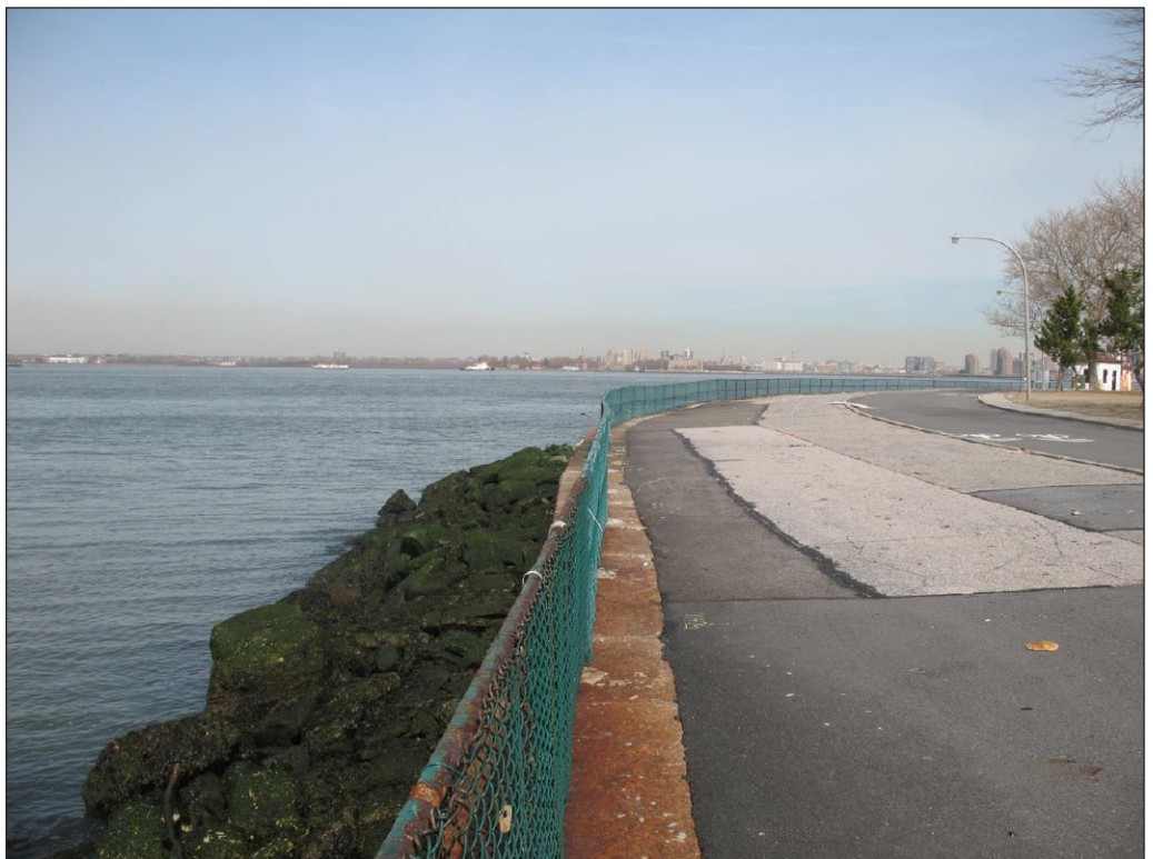
Waterfront esplanade and seawall, at Picnic Point 26
