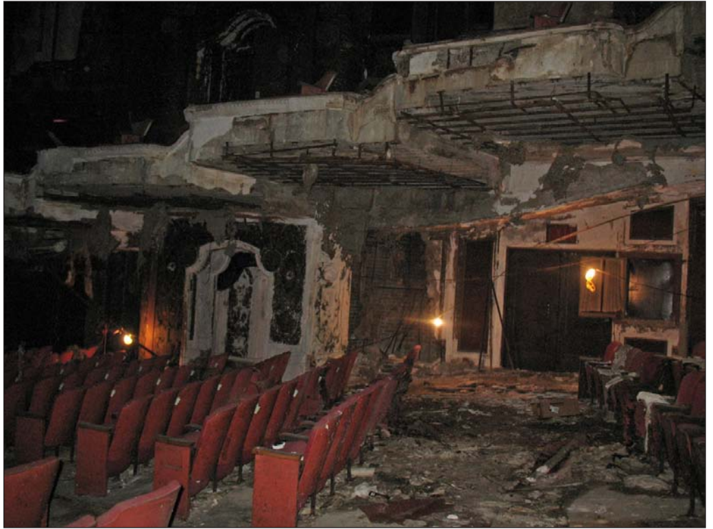
Kings Theatre, Auditorium 1e
