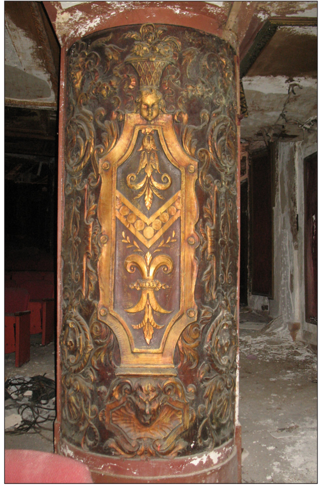
Kings Theatre, Auditorium column 1c
