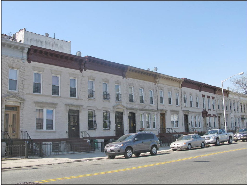
Ten Rowhouses on south side of Beverly Road between East 22nd and 23rd Streets 9
