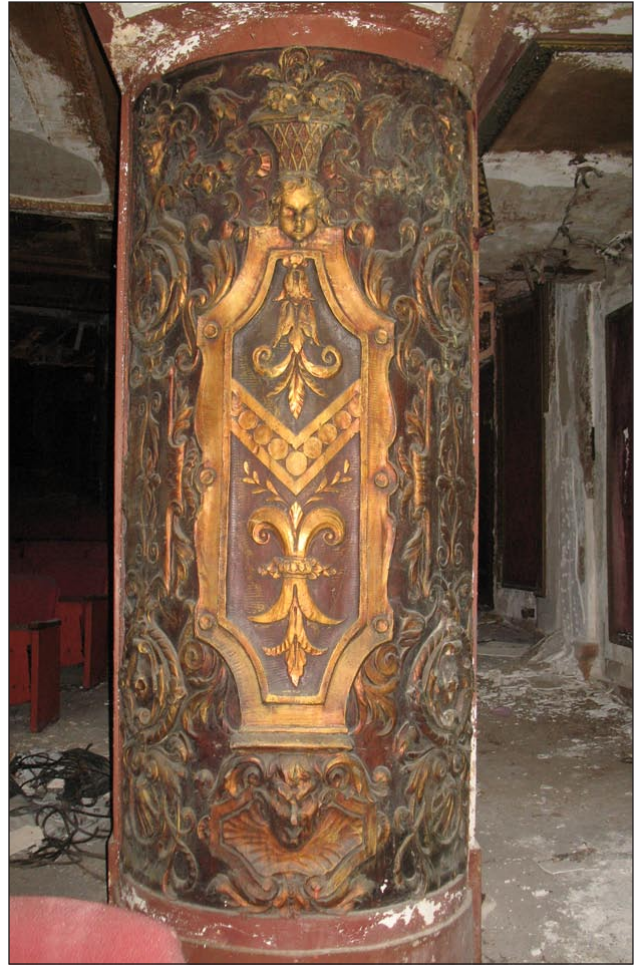
Kings Theatre, Auditorium column 1c
