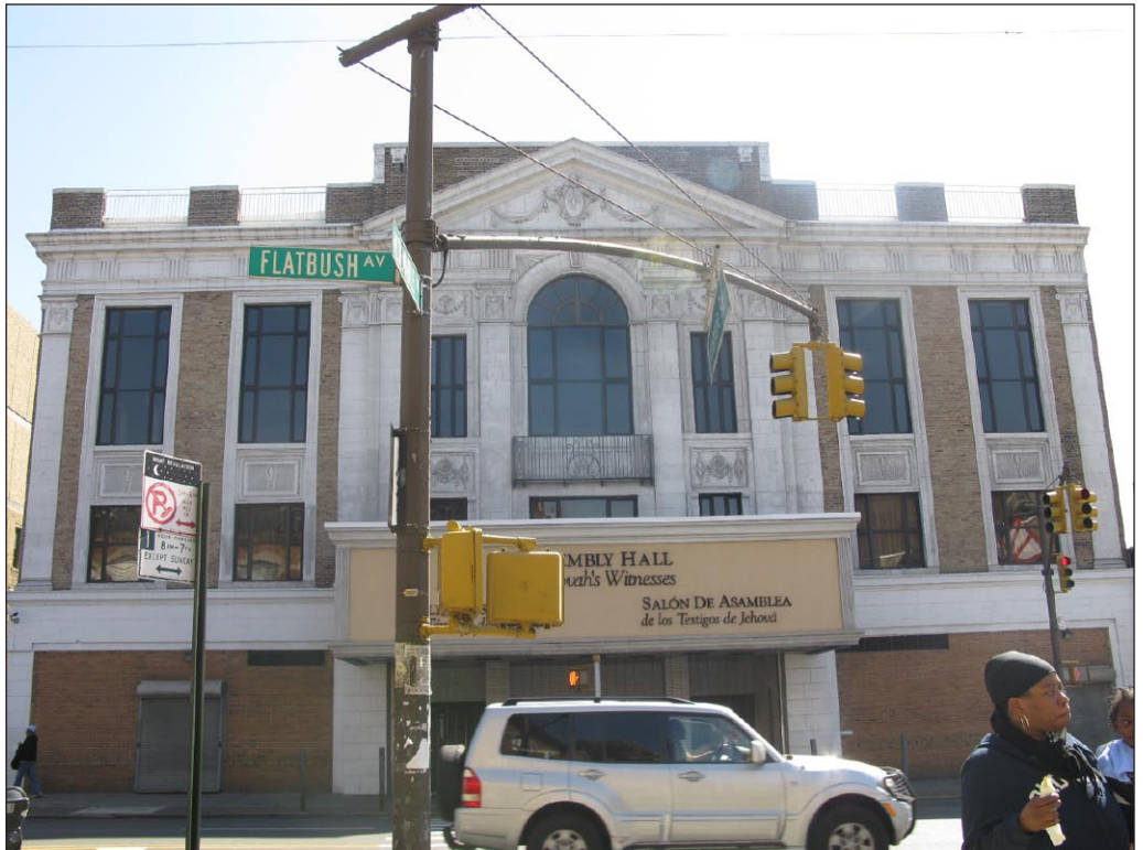
Former Albemarle Theater, 977 Flatbush Avenue 5
