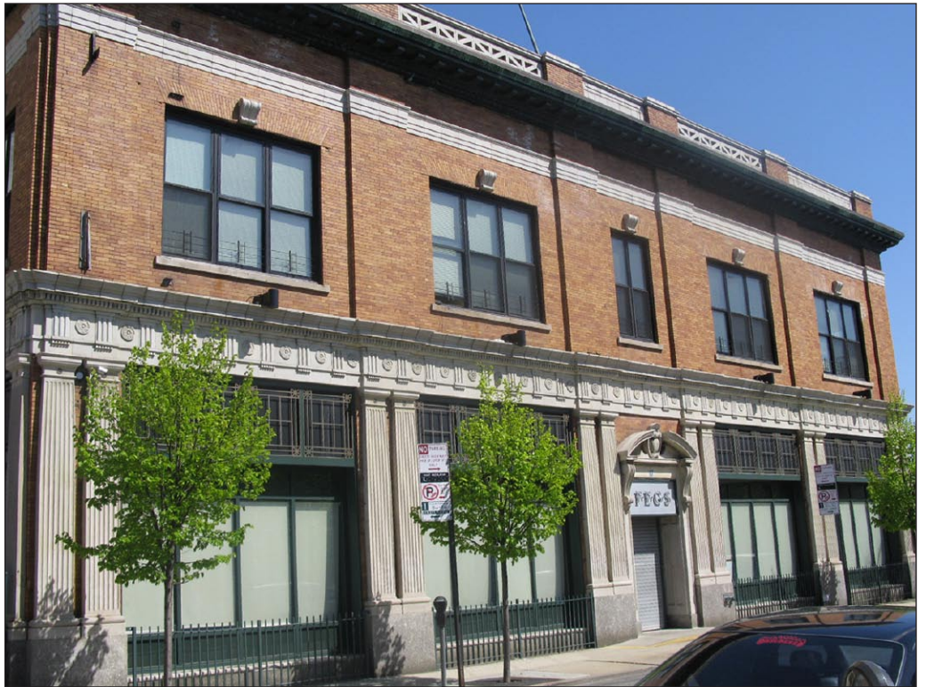
Former Brooklyn Union Gas Company, 19 Duryea Place 2
