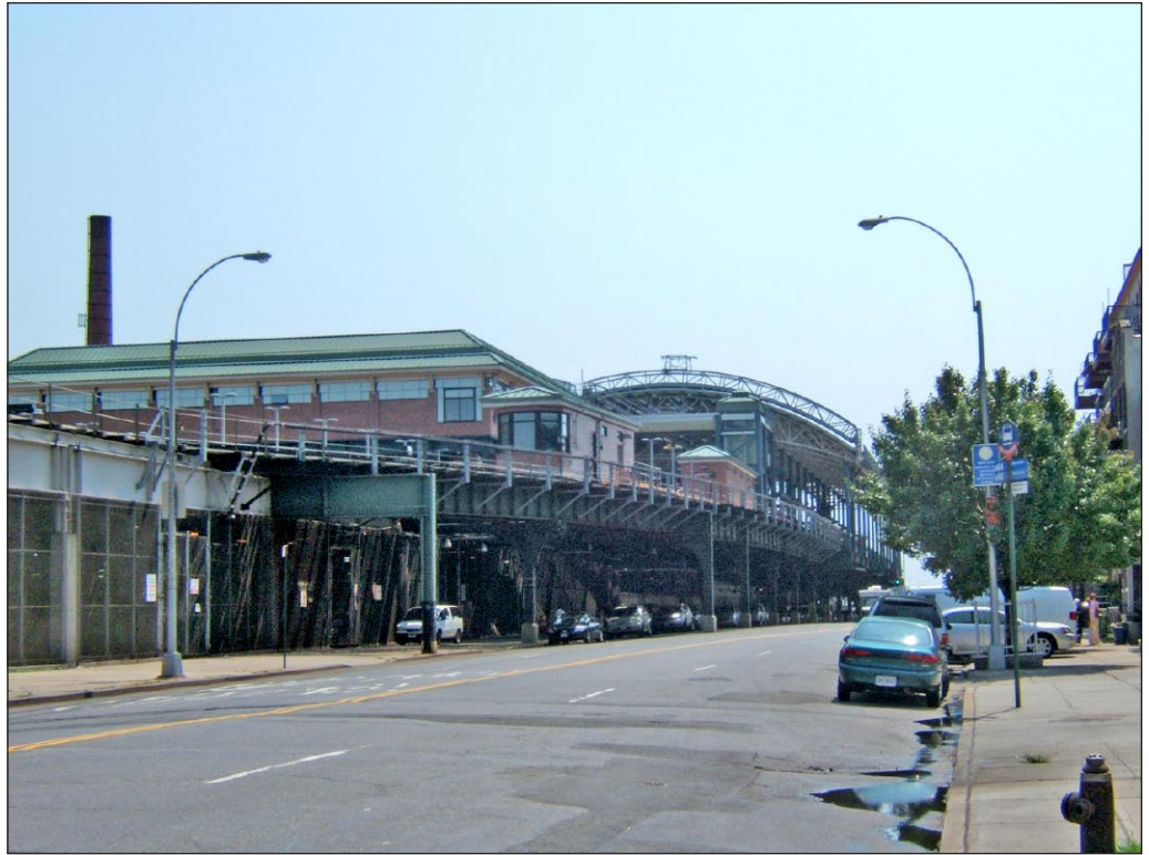
View south of the Stillwell Avenue Station on Stillwell Avenue from Neptune Avenue 27
