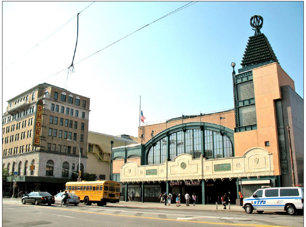
View north of Shore Theater and Stillwell Avenue Station from 23 south side of Surf Avenue east of Stillwell Avenue
