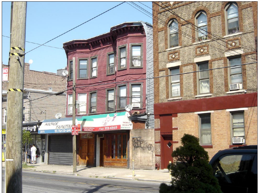
Tenements (26) at 2875-2877 West 17th Street. View east 36
