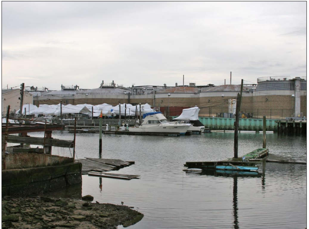
View of Coney Island Wastewater Pollution Control Plant on Shellbank Creek from east bank 20
