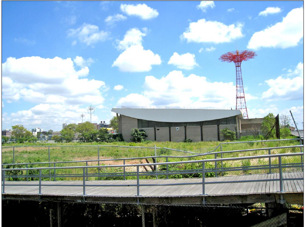
View east of Abe Stark Ice Skating Rink and Parachute Jump 17 from Riegelmann Boardwalk at West 21st Street
