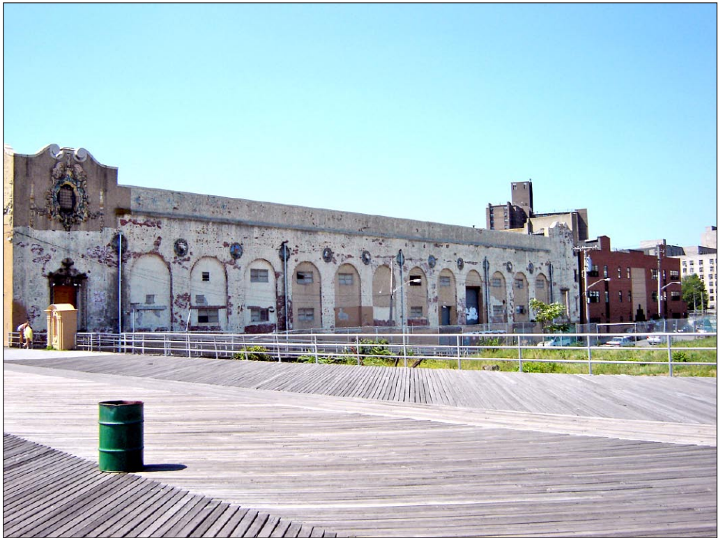
View of east façade of Childs Restaurant from Riegelmann Boardwalk near West 21st Street 16
