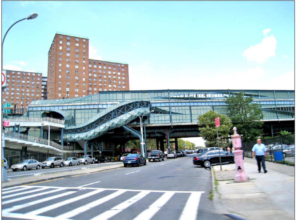
View north of the West 8th Street – NY Aquarium Subway Station 33 from Surf Avenue at West 8th Street
