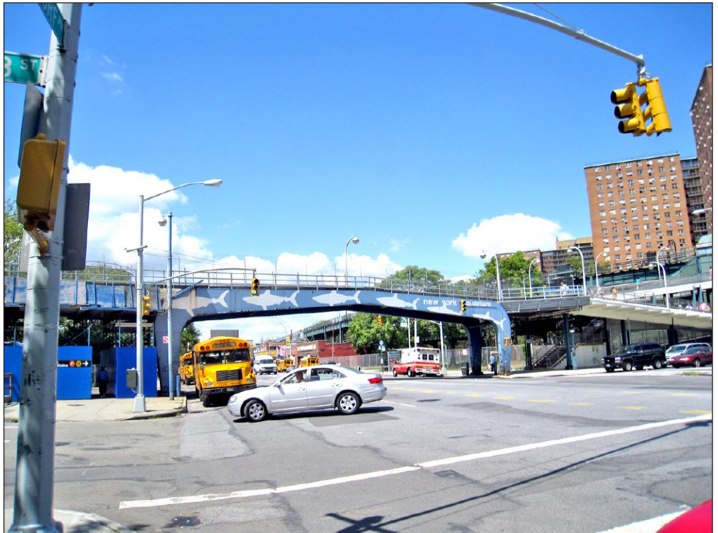
View west on Surf Avenue from West 8th Street 25
