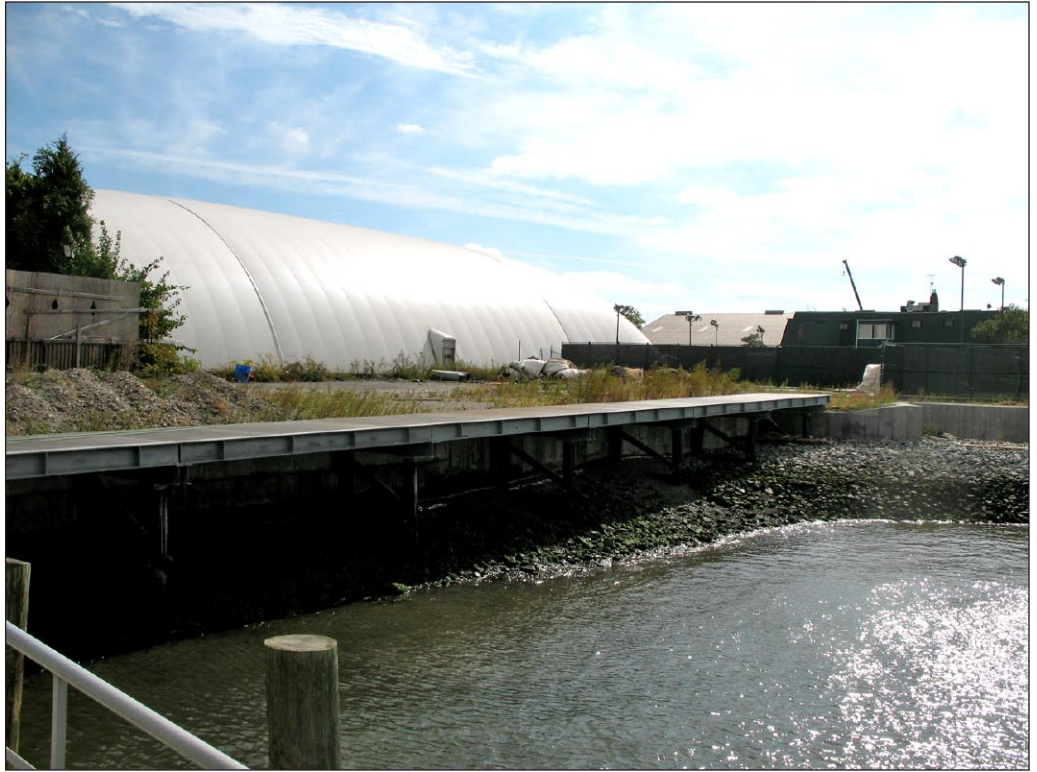
Facing south at tennis facility 1
