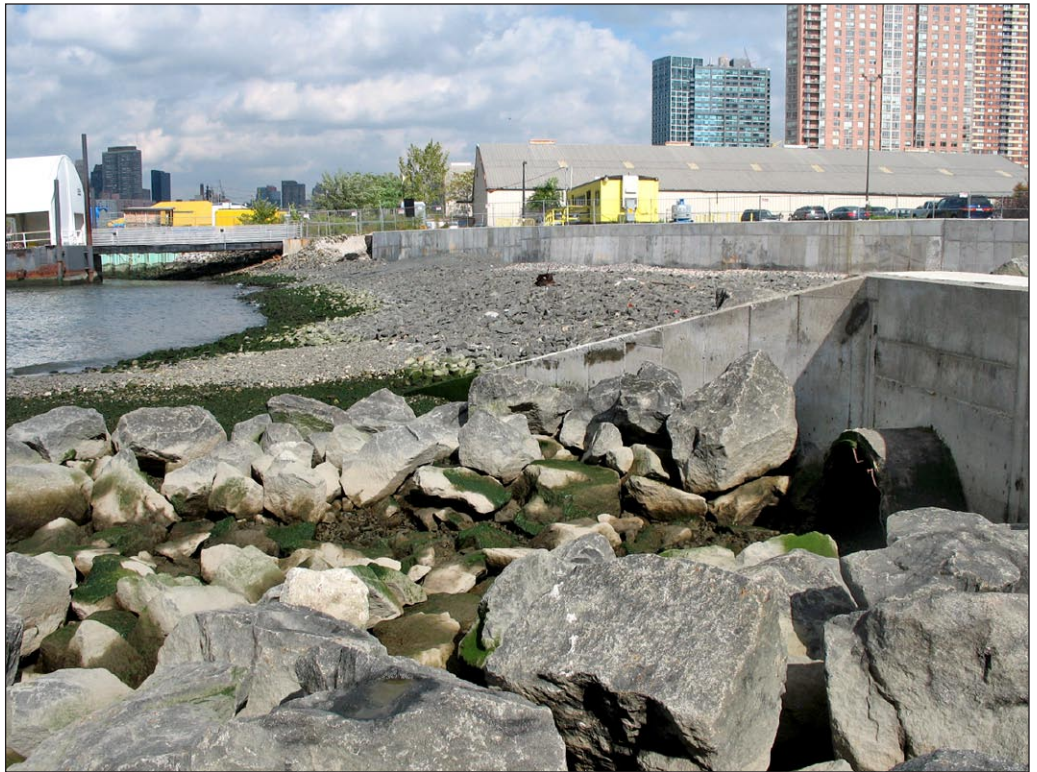
Facing north at beach area and sewer outfall to water taxi landing (low tide) 2
