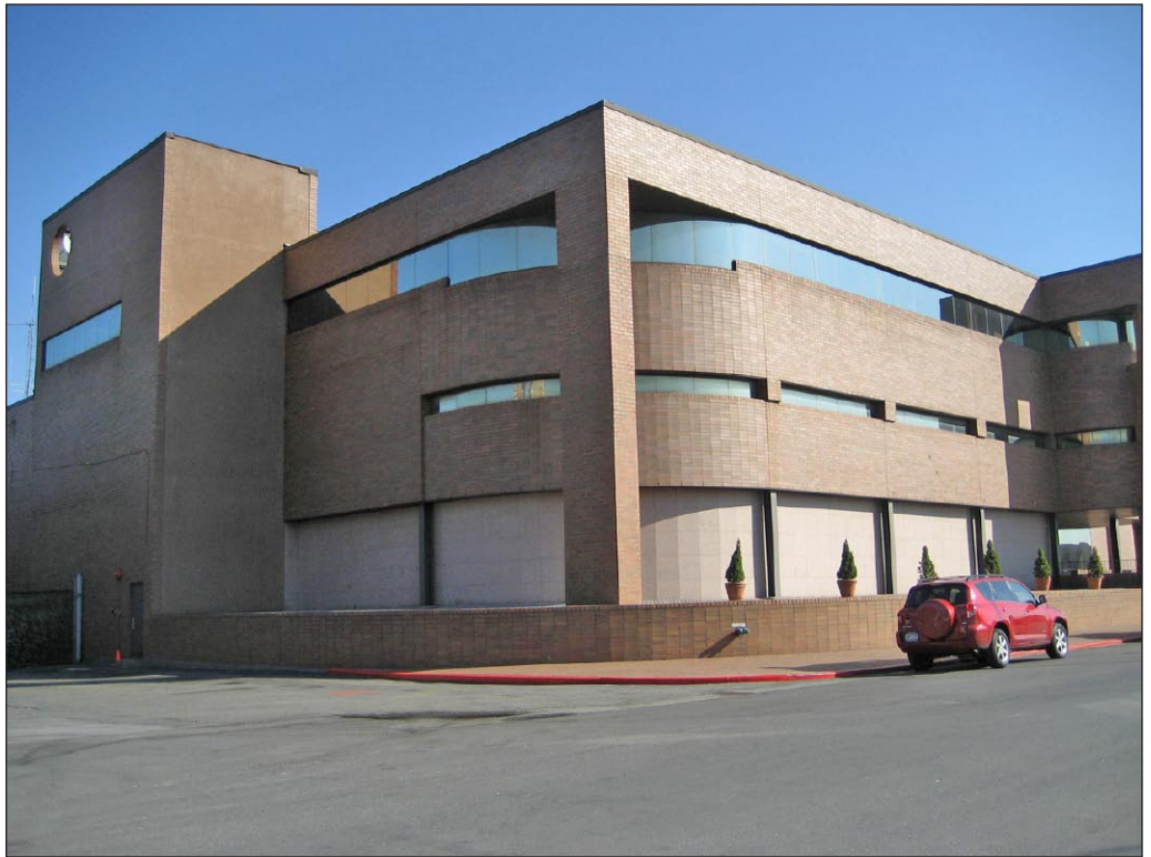
Anheuser-Busch distribution facility (Site B) looking southeast from 2nd Street 6
