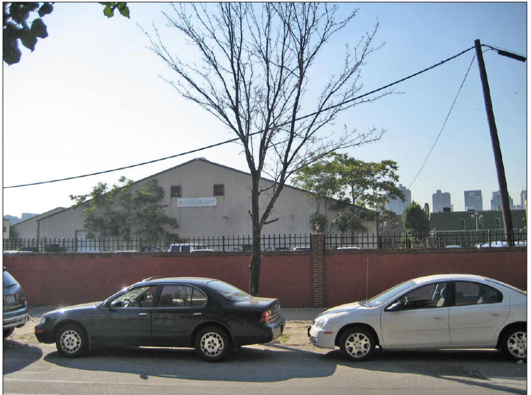
Site A, looking west from 2nd Street and Borden Avenue 1
