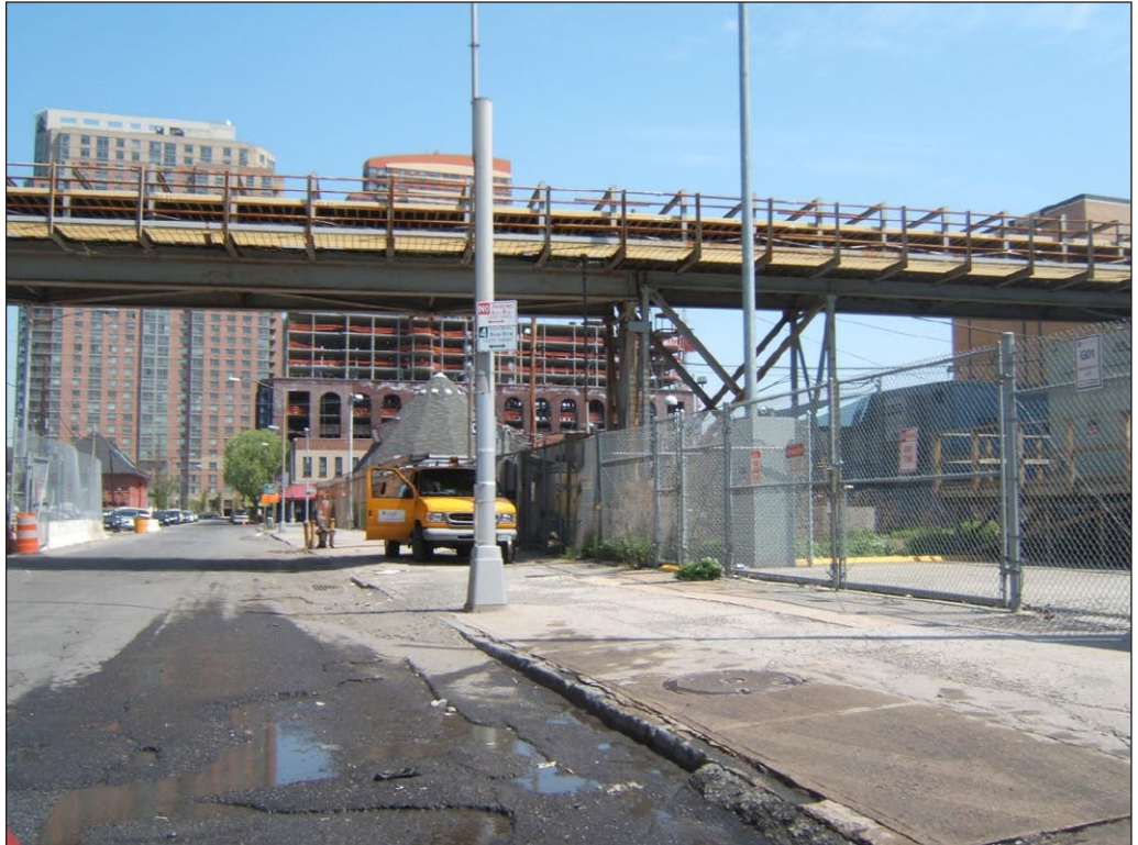
Construction bridge across 2nd Street (Site A) looking north 7
