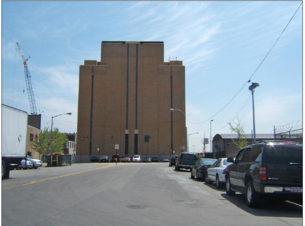
Queens-Midtown Tunnel Vent 5
