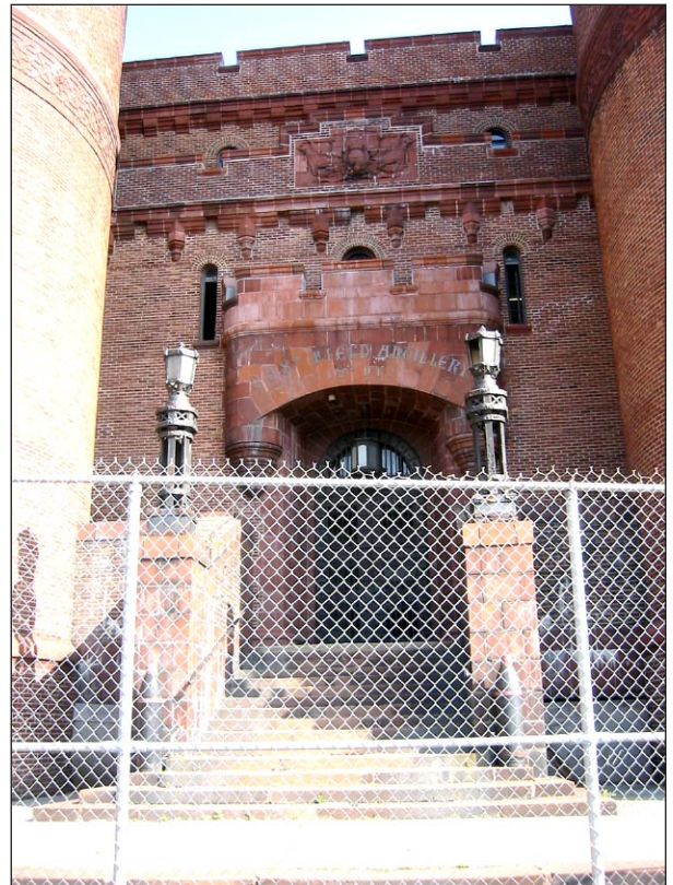
Kingsbridge Armory's primary entrance
