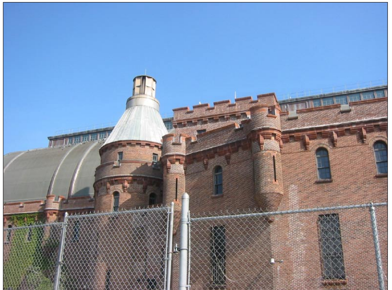
Detail of the Kingsbridge Armory's south facade 3
