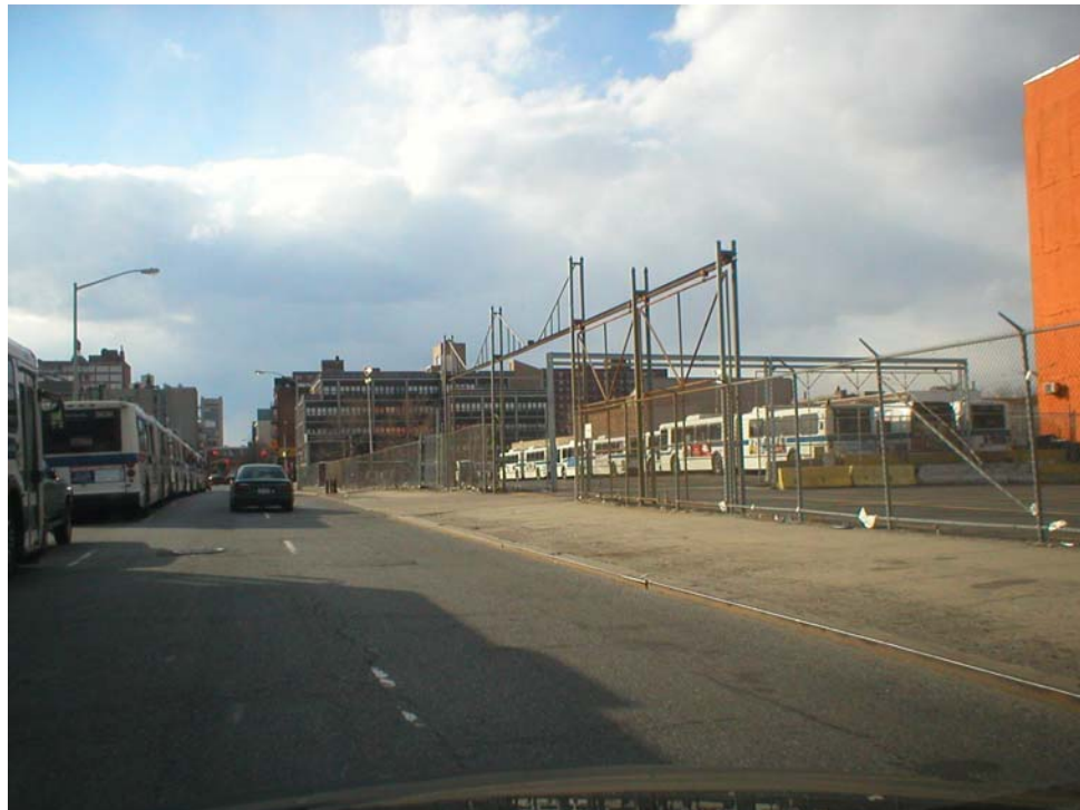
Photograph 2: View looking west on East 126 th Street with MTA bus storage on Block 1791, Lot 1.
