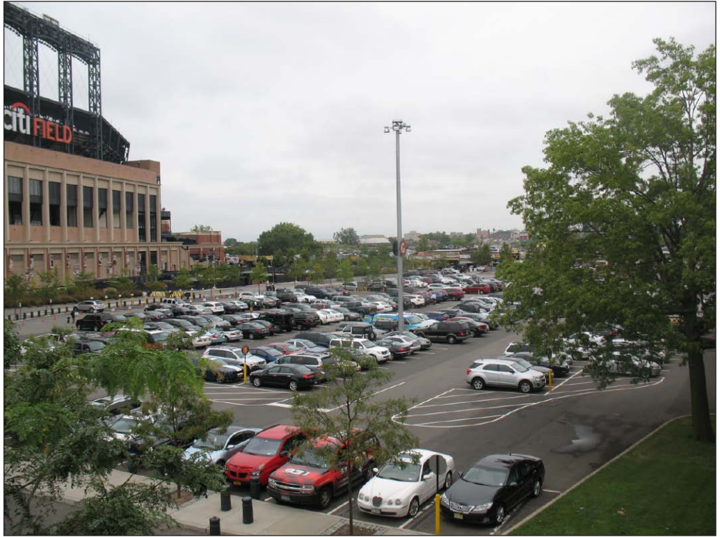
Lot B, view from No. 7 train platform 9
