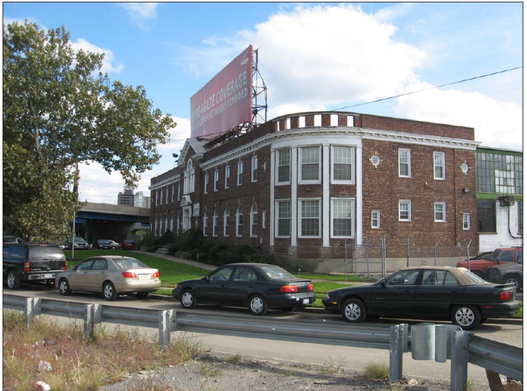
Former Empire Millwork Corporation Building 4
