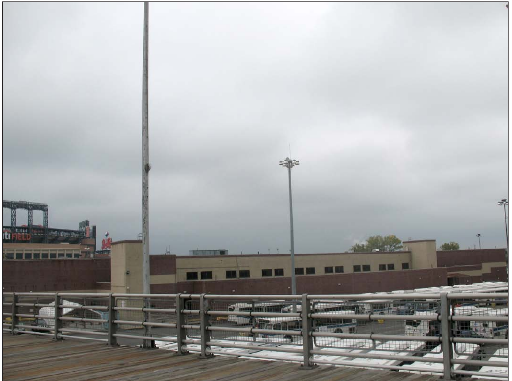
Casey Stengel Bus Depot from Passerelle Ramp 15
