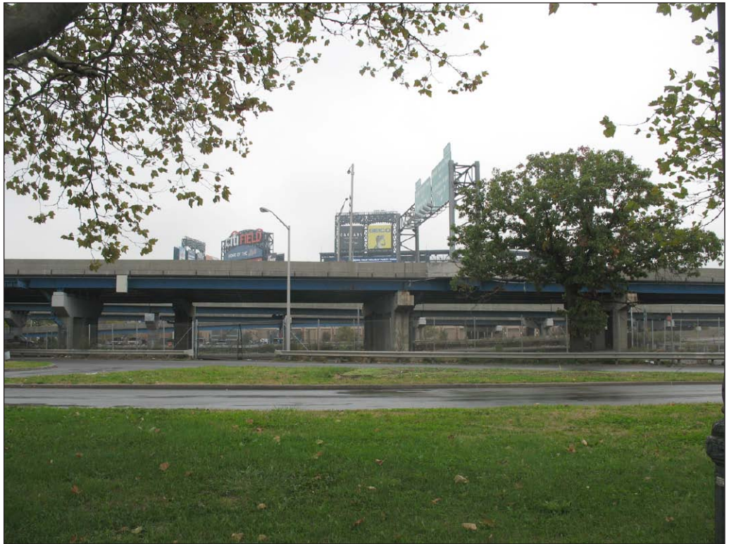
View south from Flushing Bay Promenade 10
