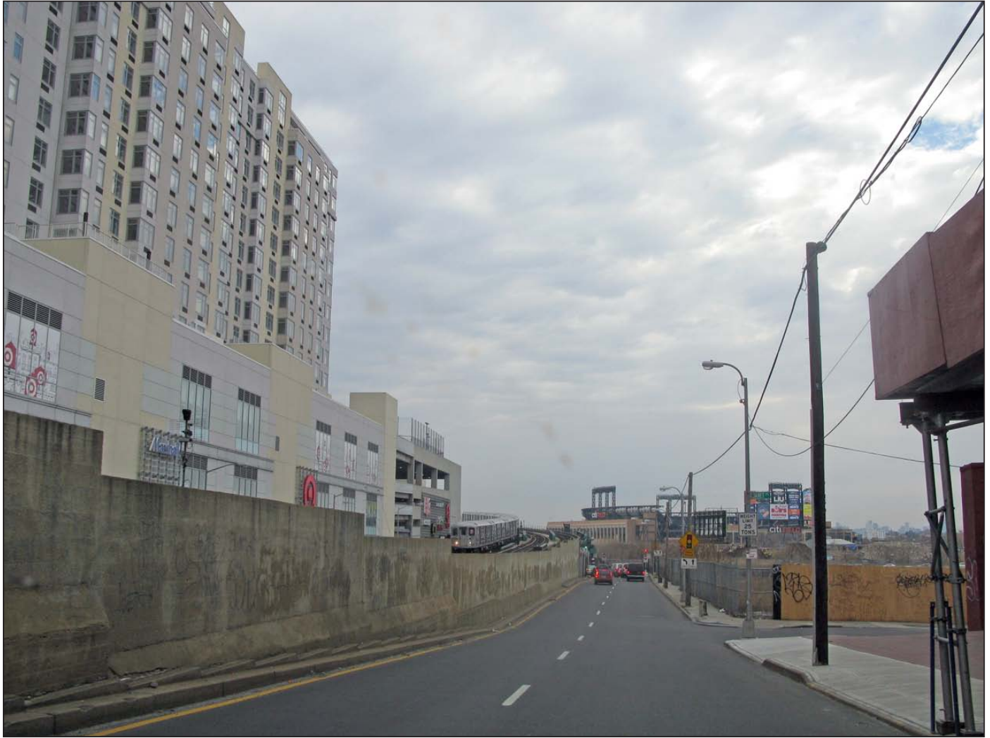
View west to project site from Roosevelt Avenue at College Point Boulevard 35
