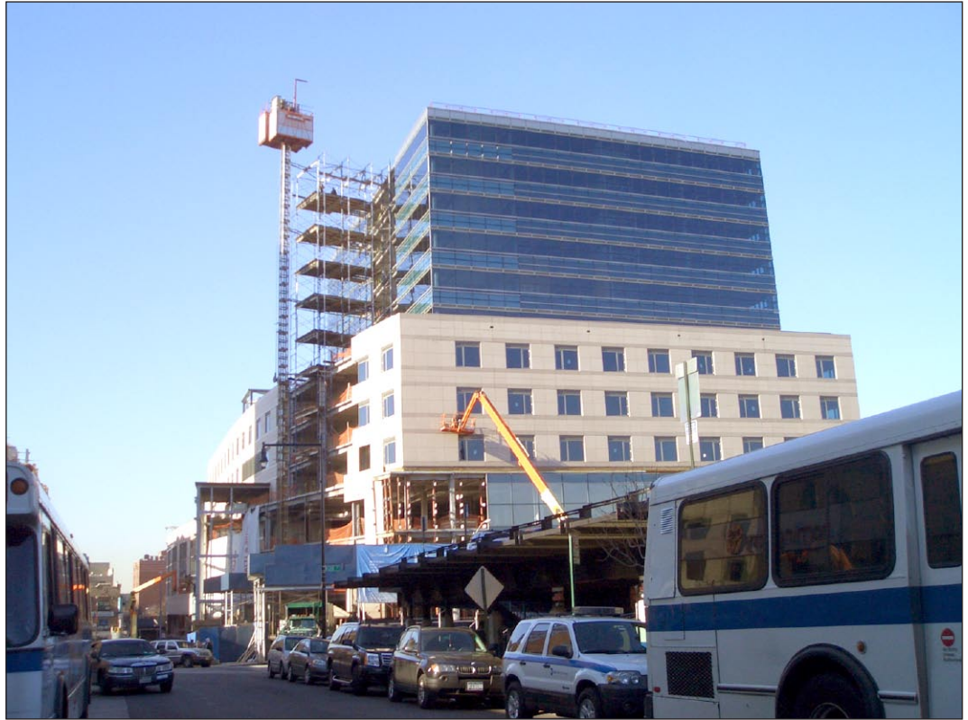
Queens Crossing development, view west along 39th Avenue from Lippman Plaza 9
