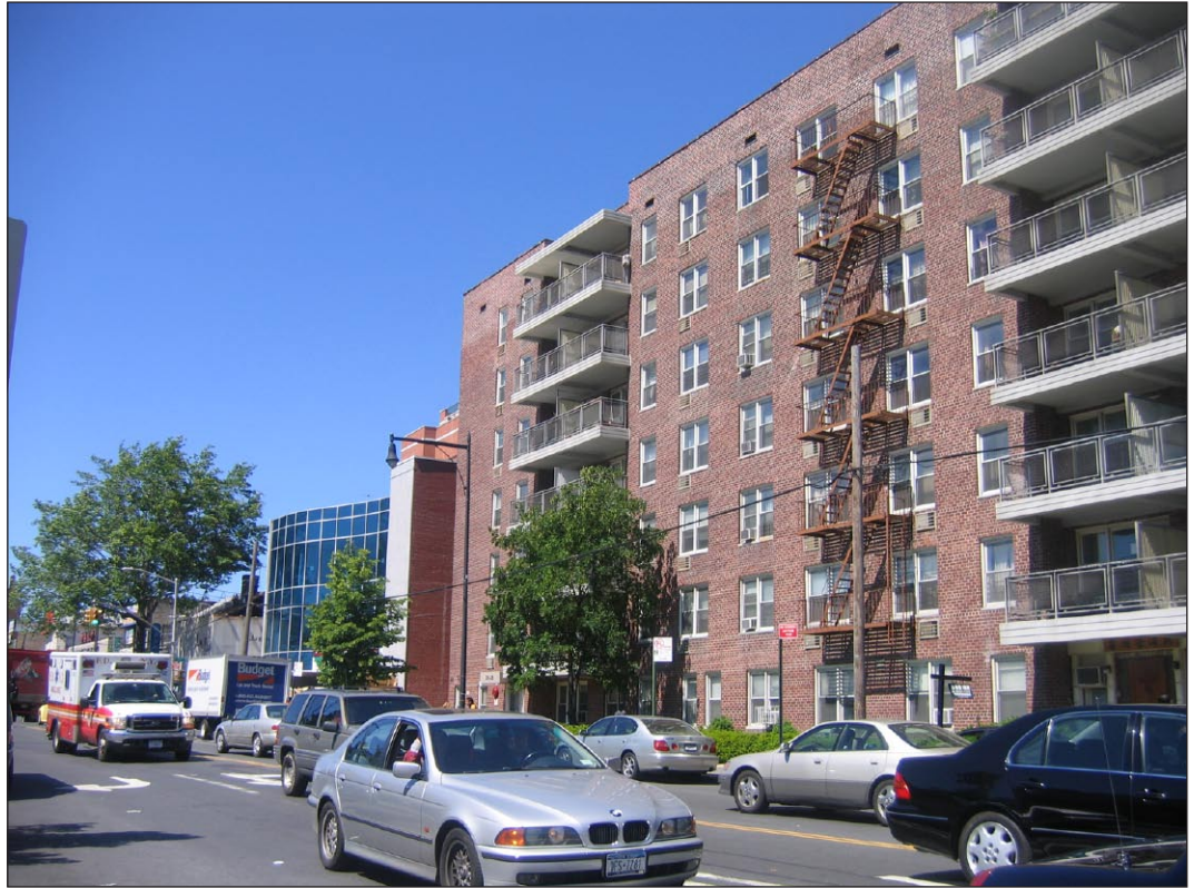
Union Street, view north from 39th Avenue 7
