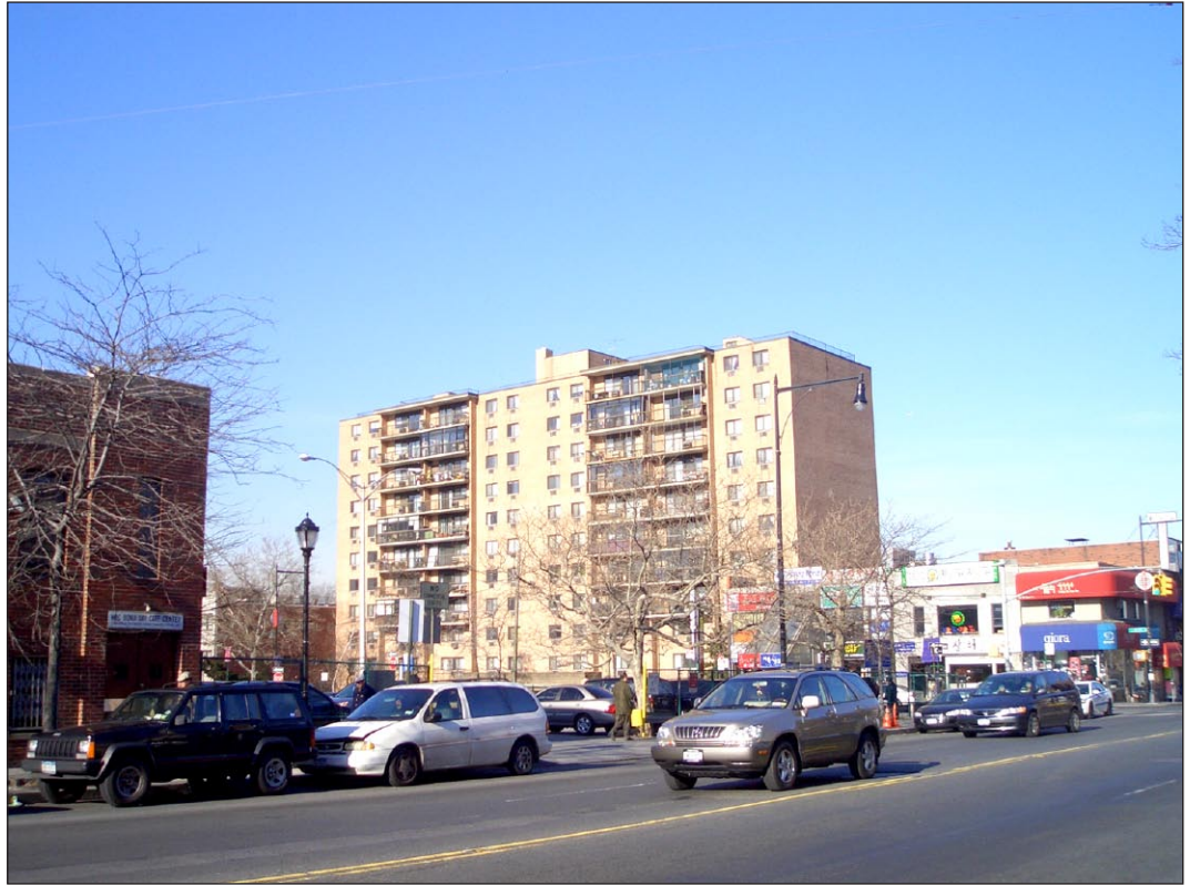
Towers Condominiums, view northwest from Union Street 11
