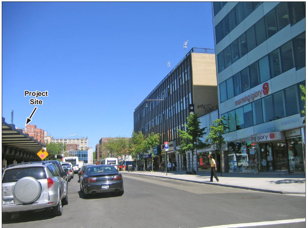
39th Avenue, view east, from 138th Street 12
