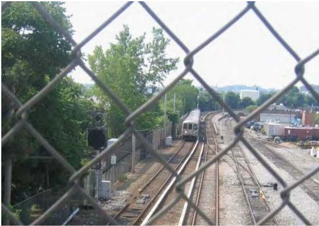
View of SIR tracks from Hannah Street.
