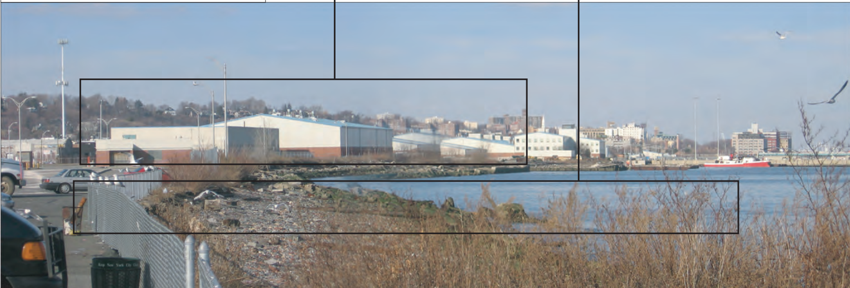
Homeport Site Shoreline | Northward View
