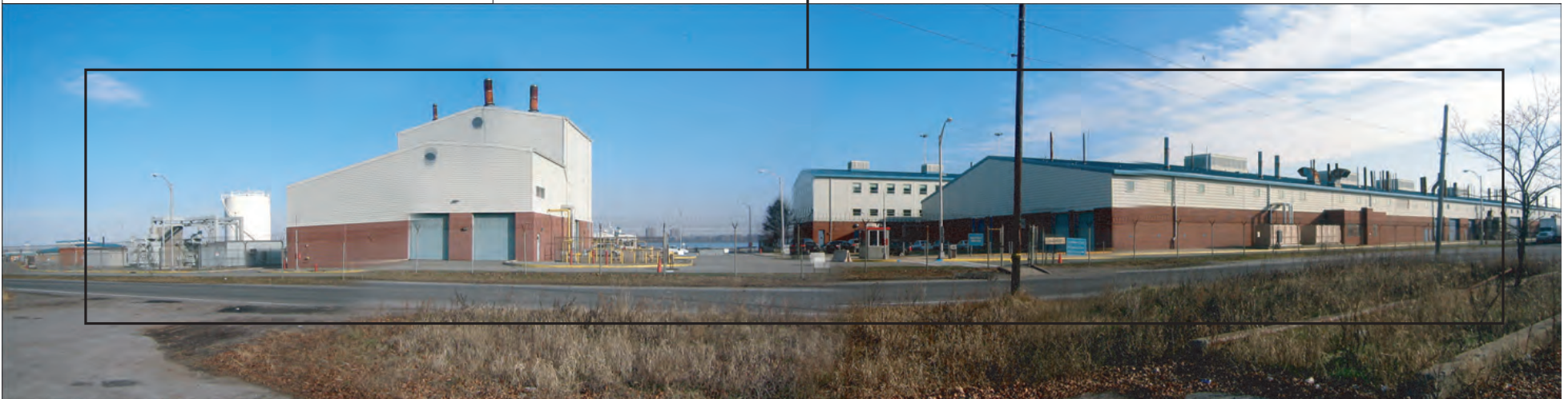
Homeport Site Buildings- Eastward View
