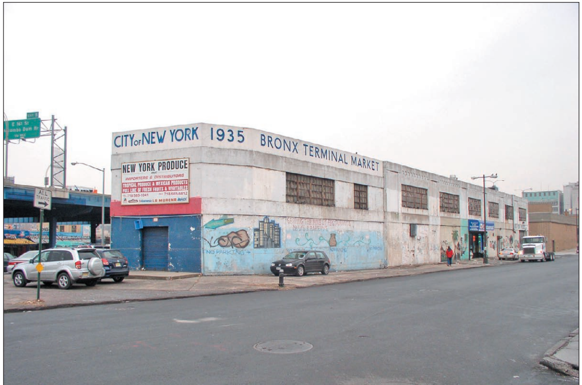
Building D, facing west from northeast corner of East 150th Street and River Avenue 4
