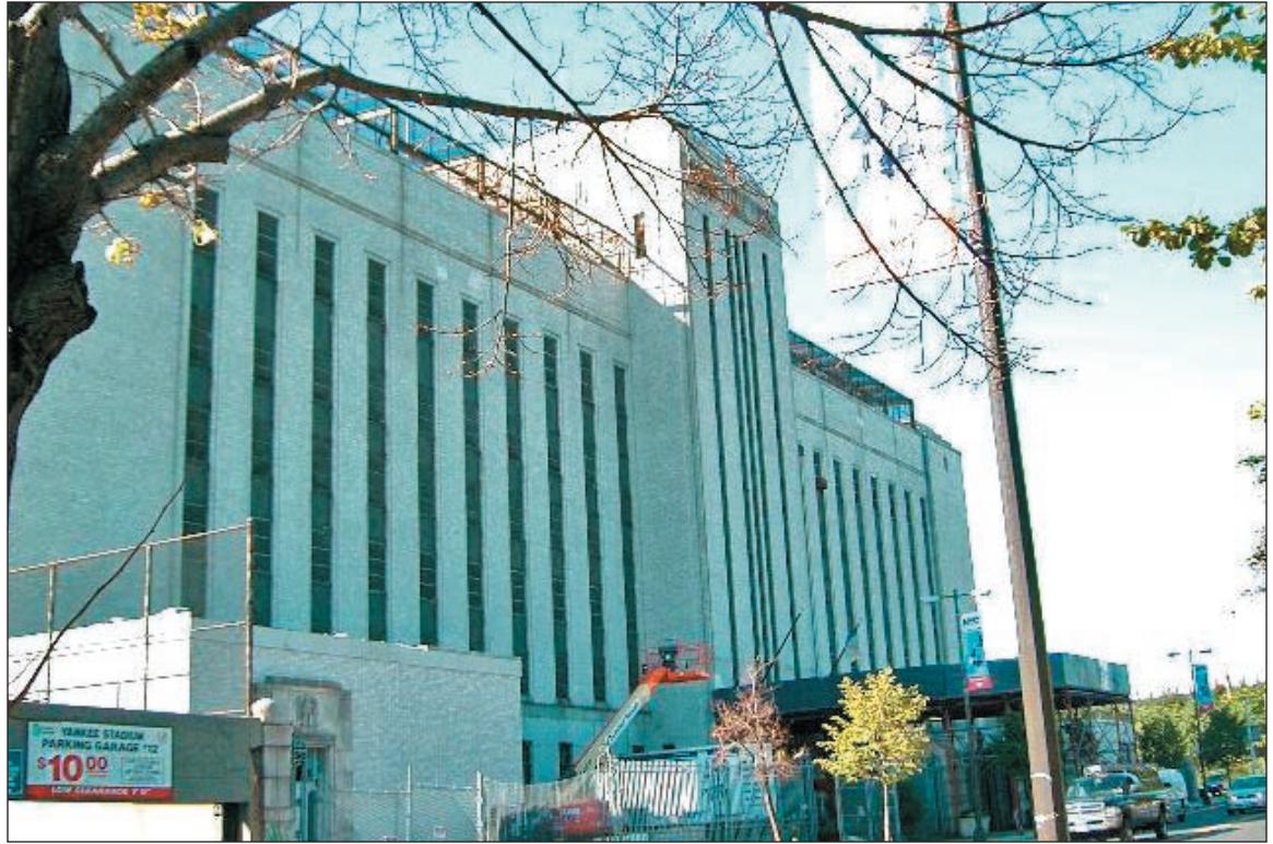
View of the Bronx House of Detention from River Avenue, facing north 1
