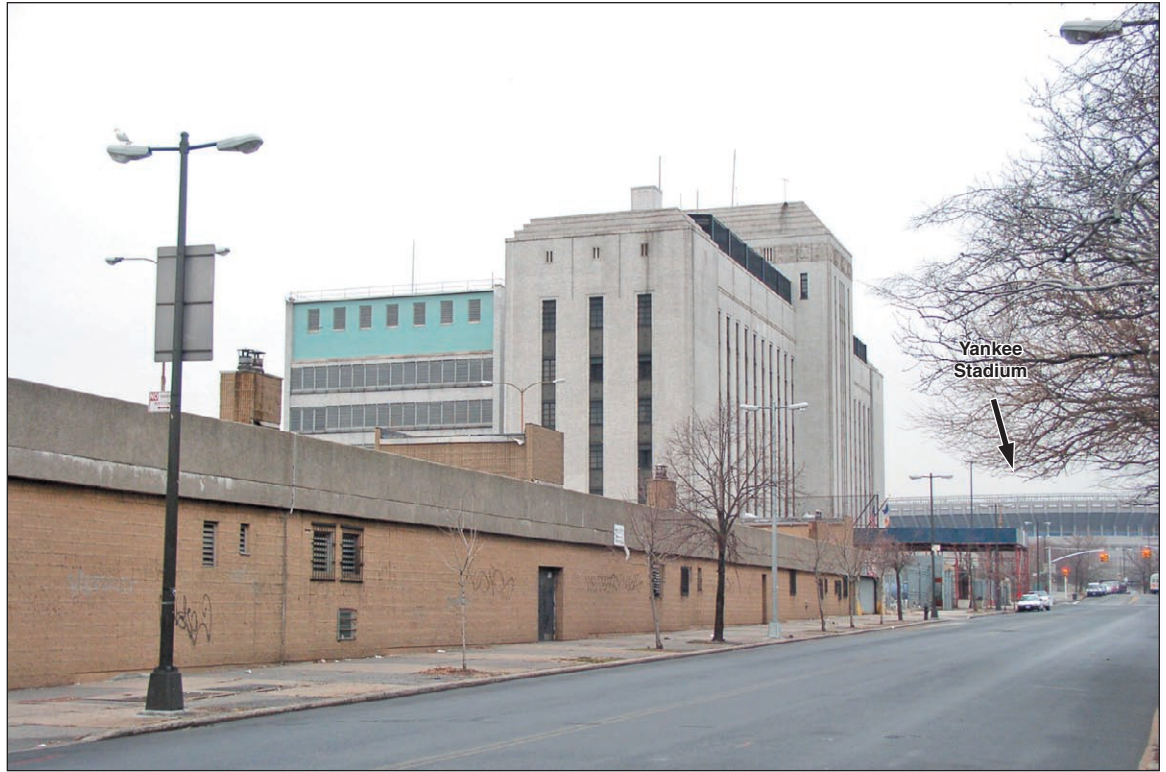
Building C and the Bronx House of Detention, view from River Avenue 5
