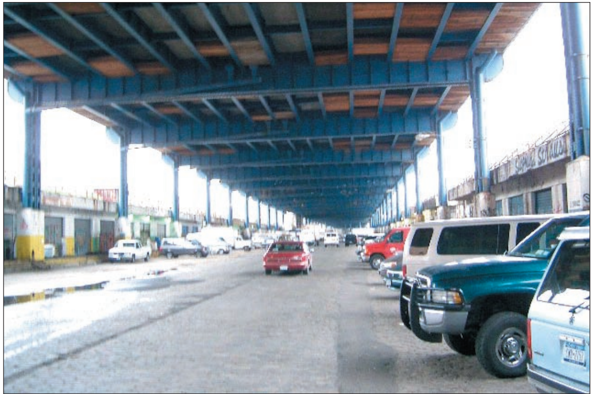
Exterior Street, view south from northern portion of project site 2
