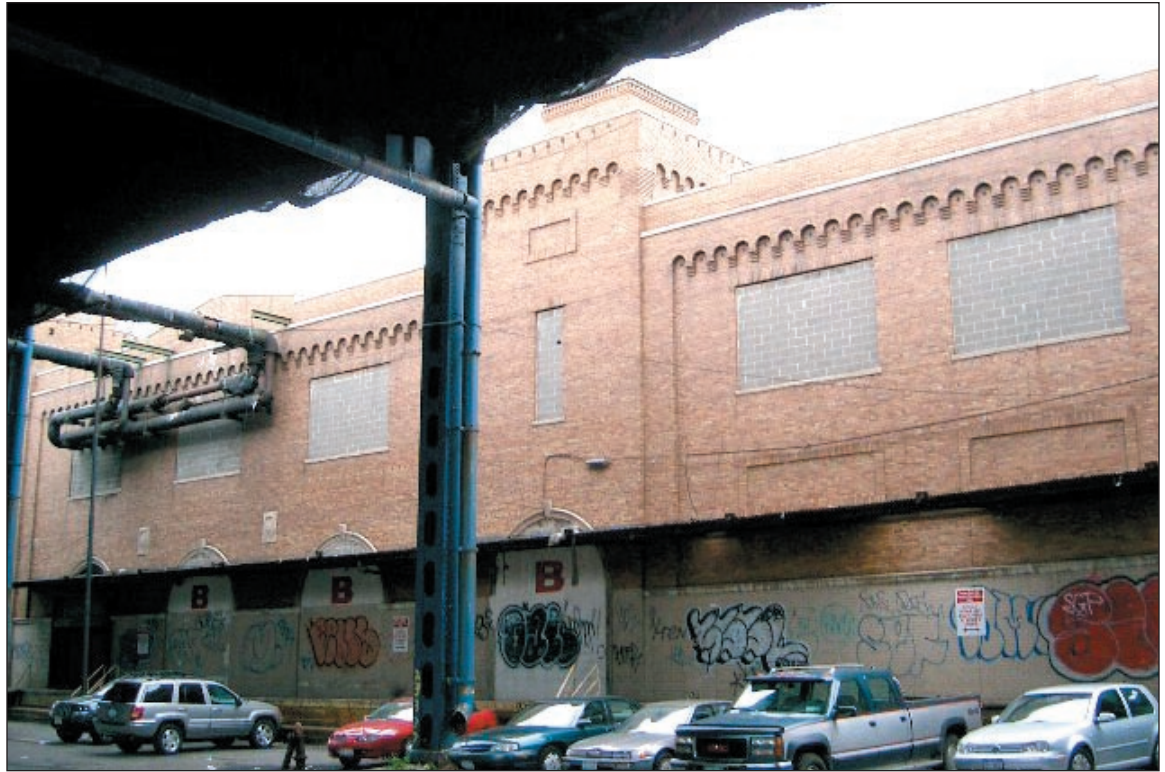
Building J, view west from Exterior Street 11
