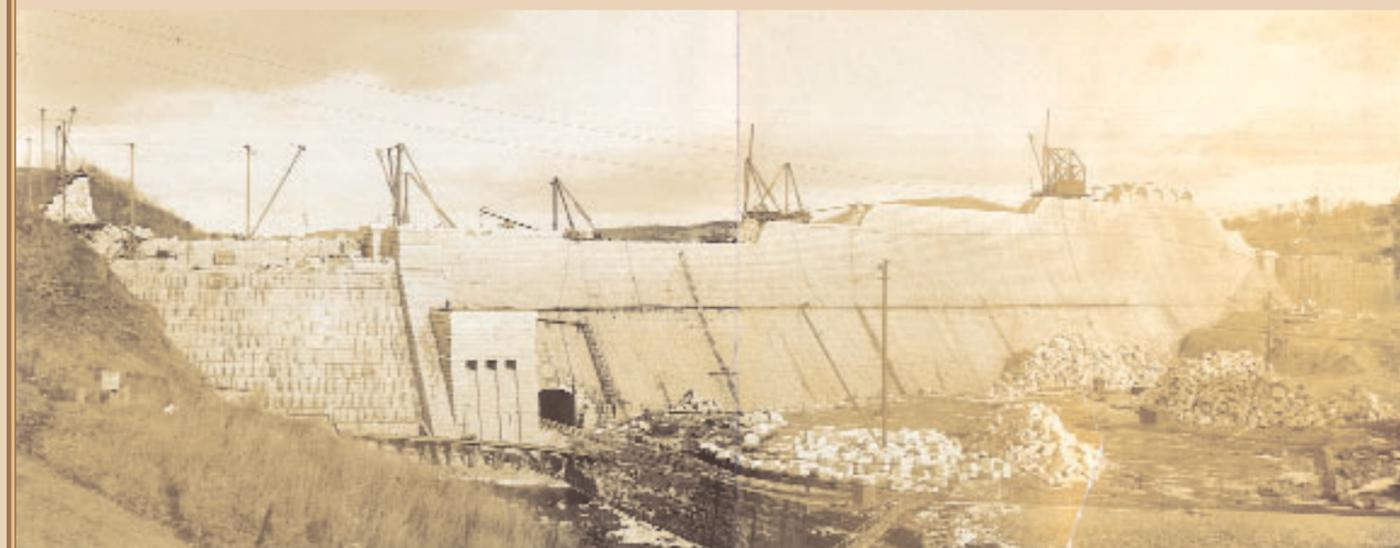
*At the height of the work, more than five hundred pieces of heavy machinery were operating on the site, and 1,500 men were on the payroll. Some 745,000 barrels of cement would be used, and 100,000 tons of coal kept the machinery operating.*
