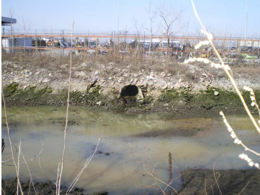
Site Photograph 5-8: Outfall into drainage ditch from western portion of NYPD Tow Pound.
