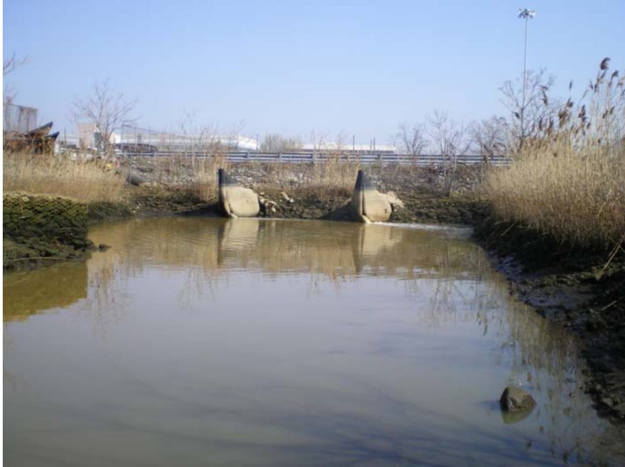
Site Photograph 5-4: Looking north at the northern crossing of drainage ditch. Note attached tide gates.
