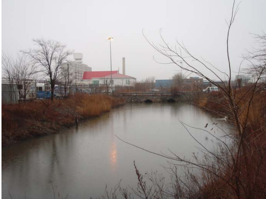
Site Photograph 5-6: Drainage ditch at the 90 degree bend looking south at northern crossing.
