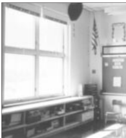
Low-e, high performance glass improves the efficiency of this school's windows. The fixed casement and awning units, installed by Andersen Windows, also open to let in fresh air.
