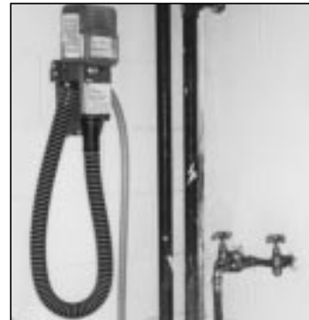
Dilution systems, such as this, for concentrated cleaning products reduce solid waste generation.
