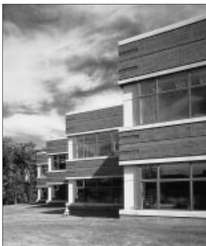
Anderson Windows installed energy efficient low-e, high performance windows at this B.F. Goodrich manufacturing facility. The fixed casement and awning units also open to let in fresh air.
