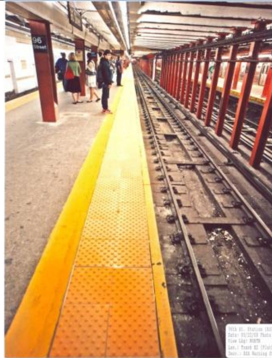
Restored Platform Edge with Tactile Tiles
