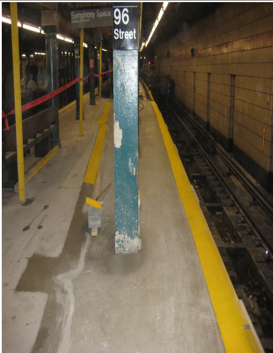
Restored Platform Edge with Tactile Tiles
