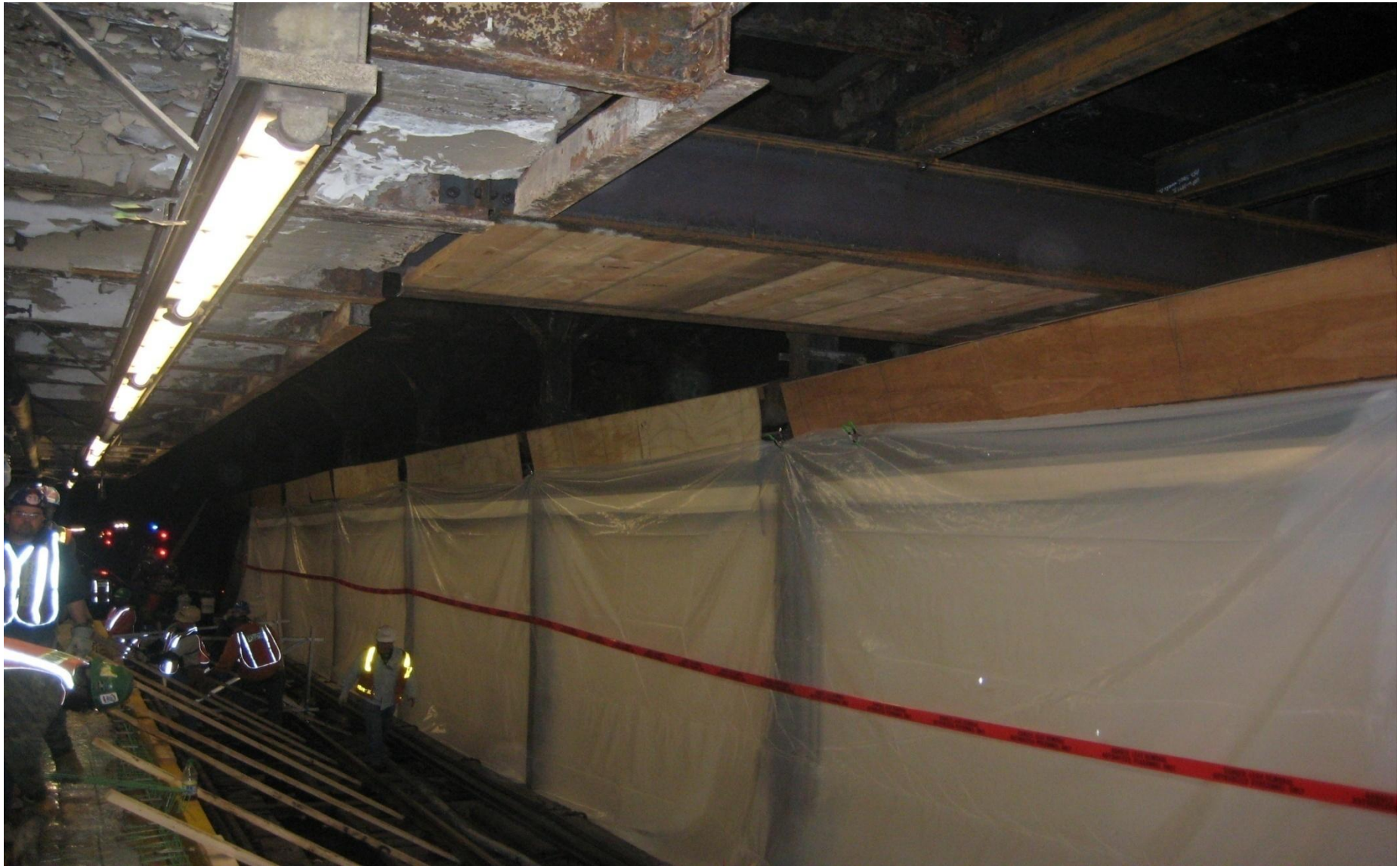
Installation of Rubbing Board and Restoration of Track Ceiling
