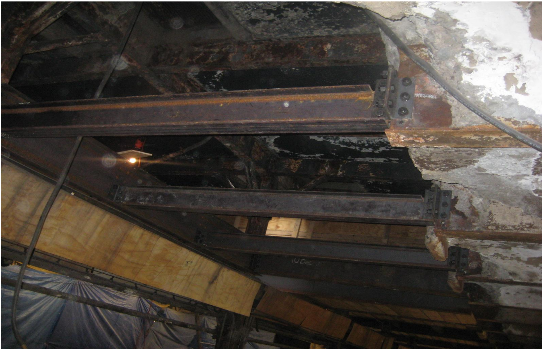
Installation of Beams & Girder for the New Track Roof
