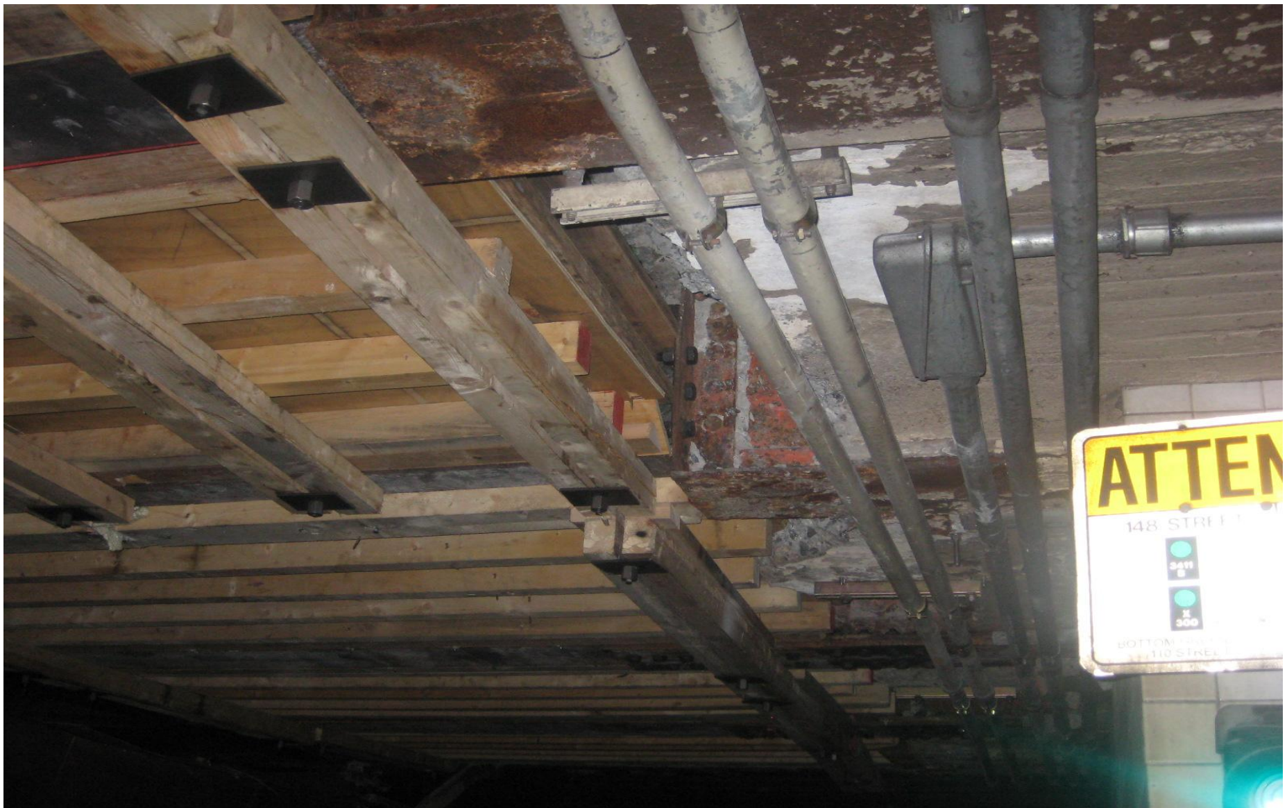
Form for Concrete Pour for Track Ceiling Roof
